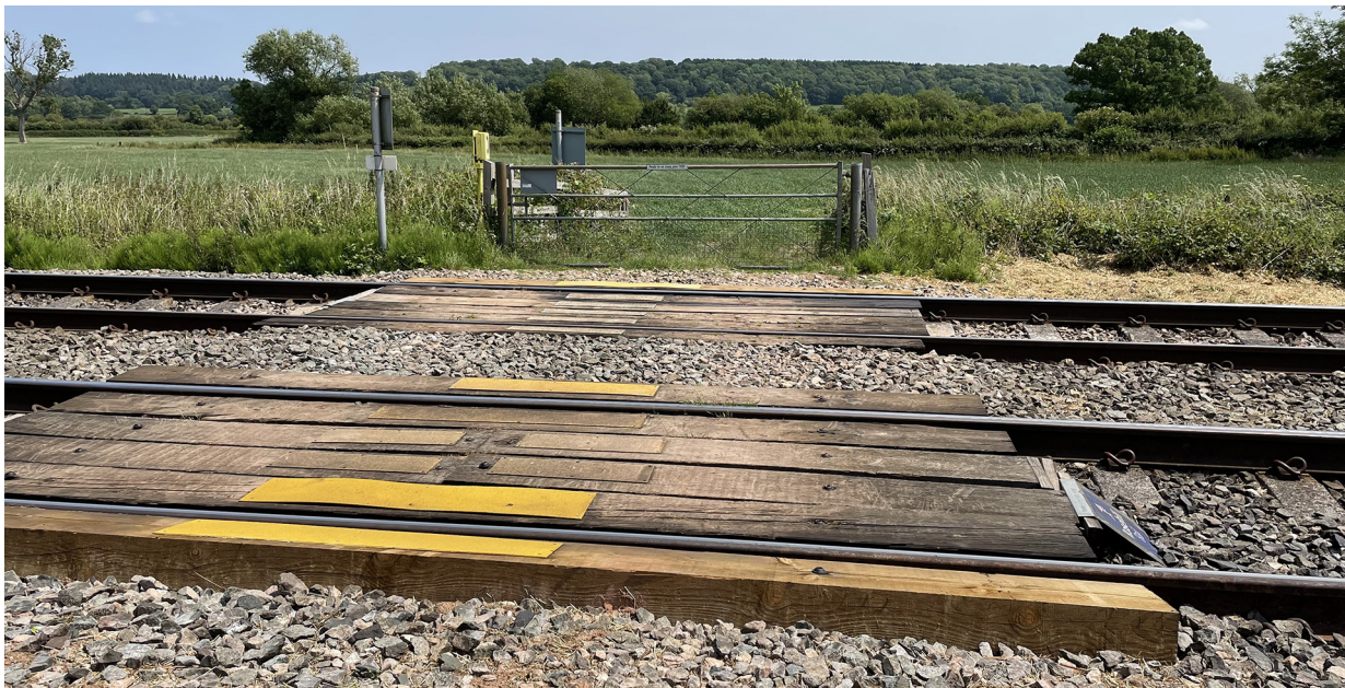
Figure 5: Nordan Farm level crossing, including repair work done after the accident.
