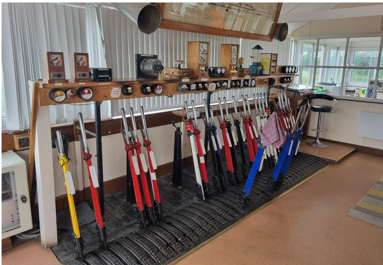
Figure 7: Interior of Woofferton signal box.
