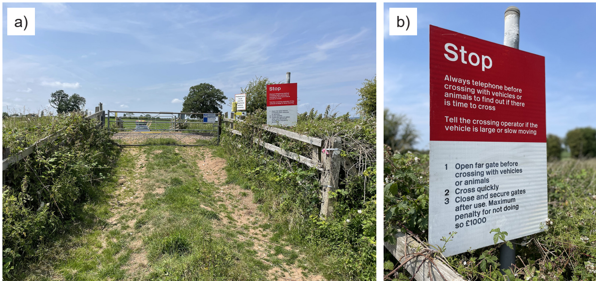
Figure 4: Approach to Nordan Farm UWC(T) from the east showing a) the general signage arrangements and b) the sign with instructions to use the crossing.
