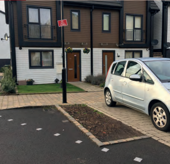
203 Landscaping between car parking spaces need some vertical protection to help establish planting.
