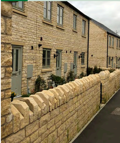
197 Boundary treatments can be a key way to reinforce local character. Also note how the meter boxes have been painted to match the facing material
