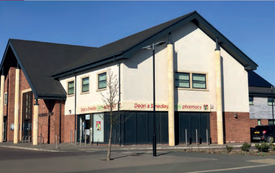
52 Active frontages are not created when windows are obscured.
