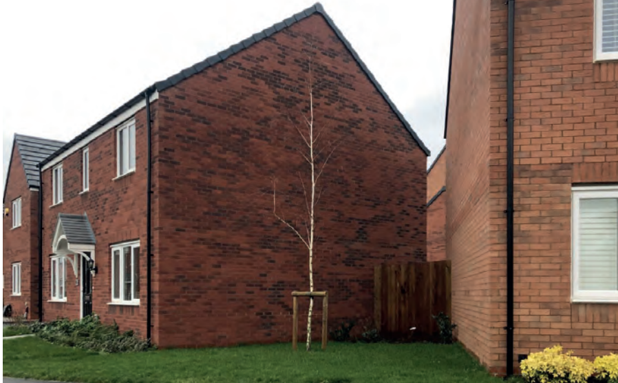
118 Blank gables are not a good way to turn a street corner.
