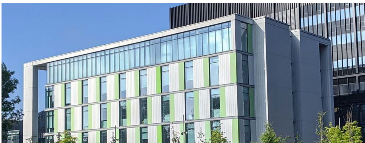
Figure 3: James Chadwick Building at the University of Manchester
