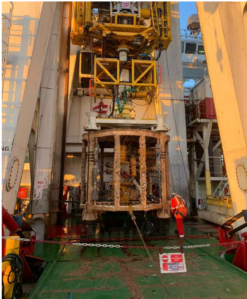
Figure 8.1.1: Protection cage recovery using WellSafe Defender
