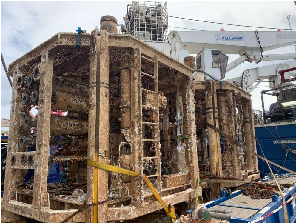
Figure 8.1.2: Protection cages recovered to back deck of vessel
