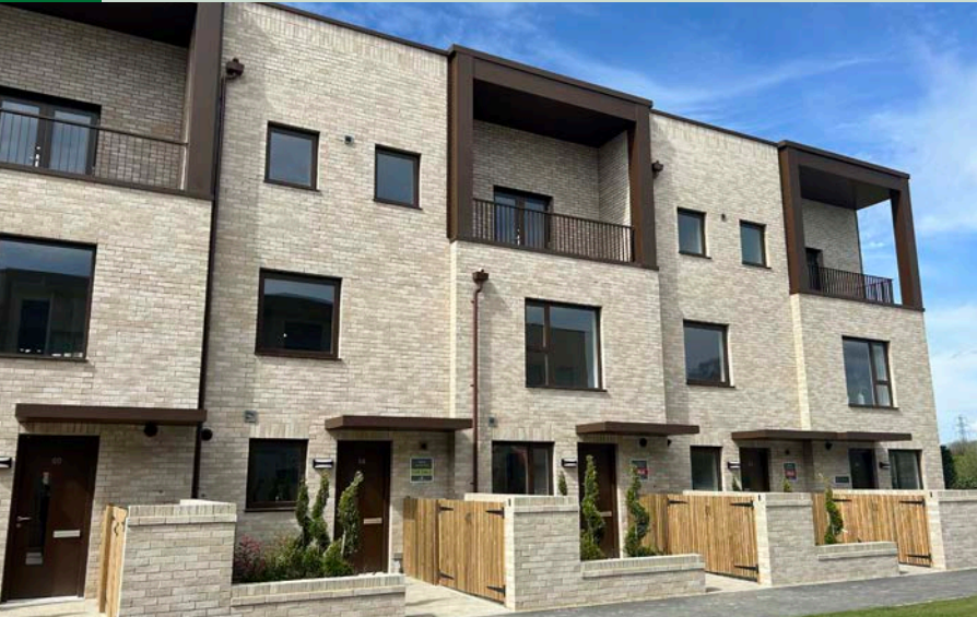
194 Town houses need a strong strategy for waste storage that is located to the front of the property.
