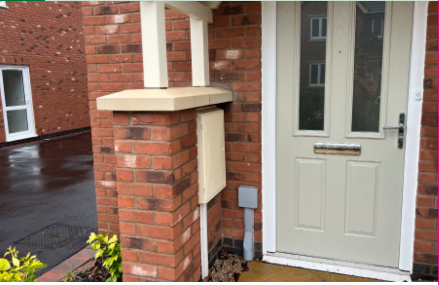
182 A utility box is better on a return wall or perpendicular to the front as it will be less visible, especially here tucked into a porch.
