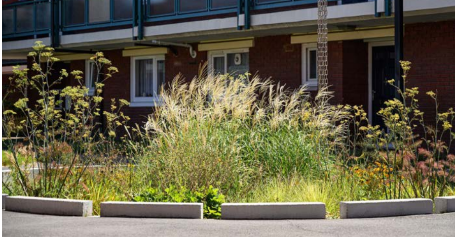
3 Manage water close to where it falls using features such as rain gardens.
