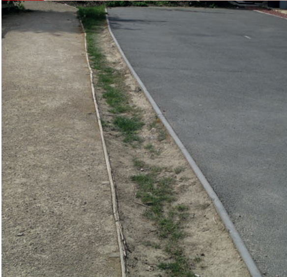
179 Narrow strips of soft landscaping between two hard surfaces will rarely take successfully.
