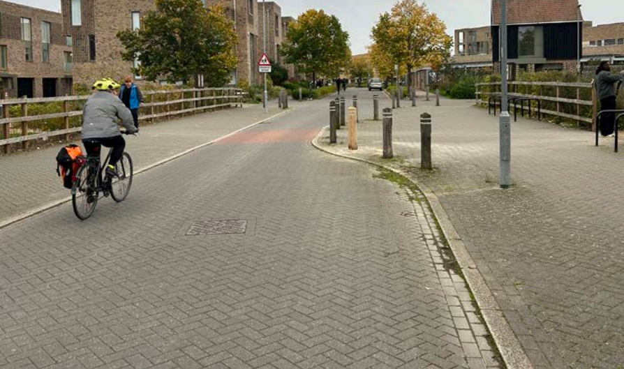
28 Slowing vehicle speeds is best done by narrowing the carriageway. Build-outs like this are better than speed ramps and can be used where people need to cross the road to access shared facilities and its safe enough to cycle on the carriageway.
