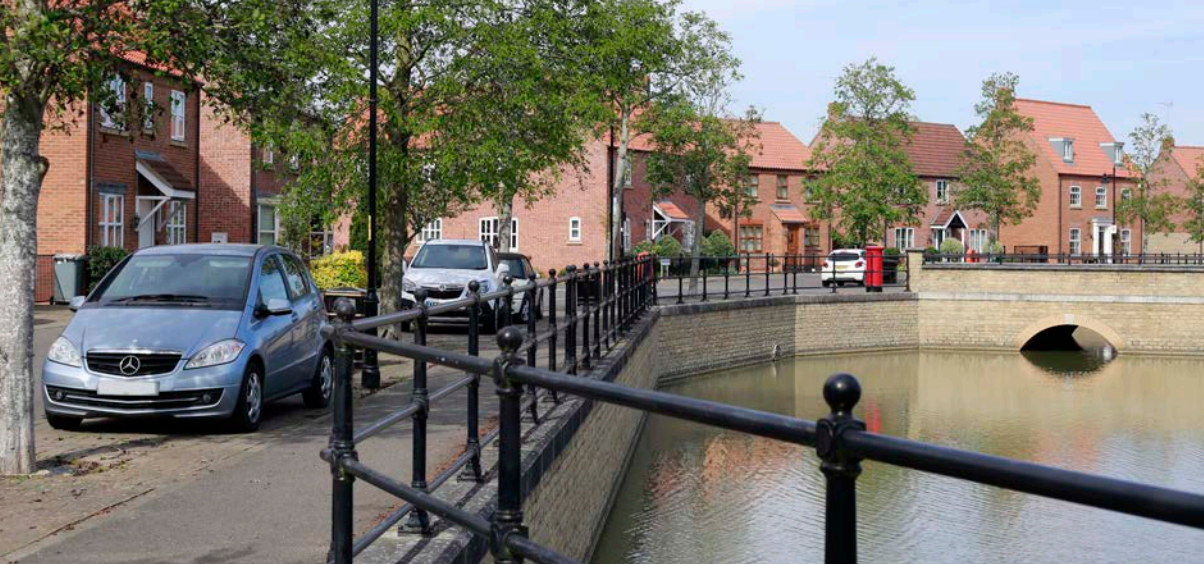
170 Attenuation basins can create spectacular spaces if afforded high quality landscape.
