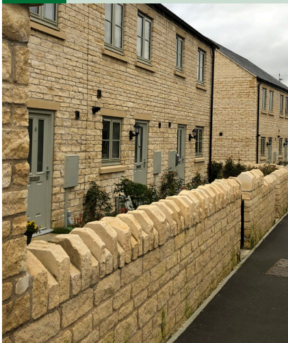
196 Boundary treatments can be a key way to reinforce local character. Also note how the meter boxes have been painted to match the facing material
