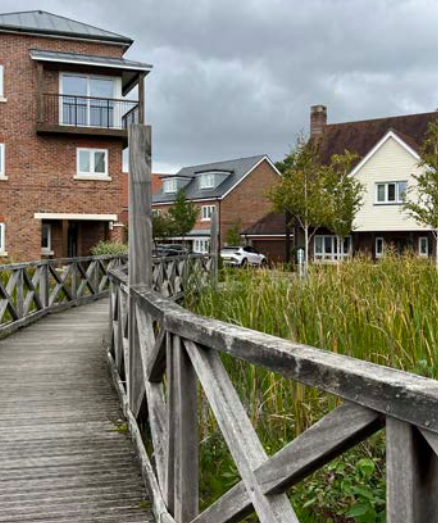
184 Projecting balconies can feel a bit exposed for residents, and overlook neighbours, but here work well overlooking the water.
