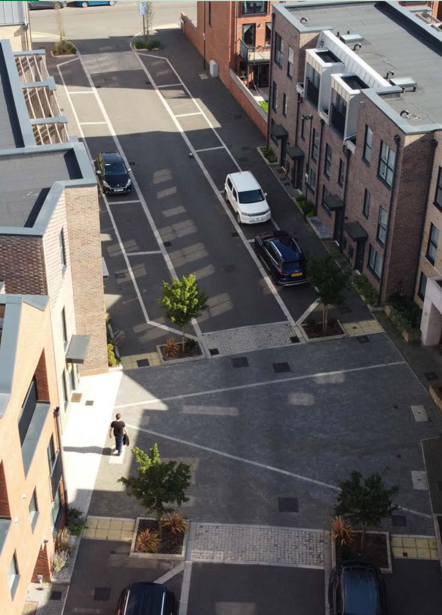
21 Variations along the street help slow cars and create streets rather than roads.
