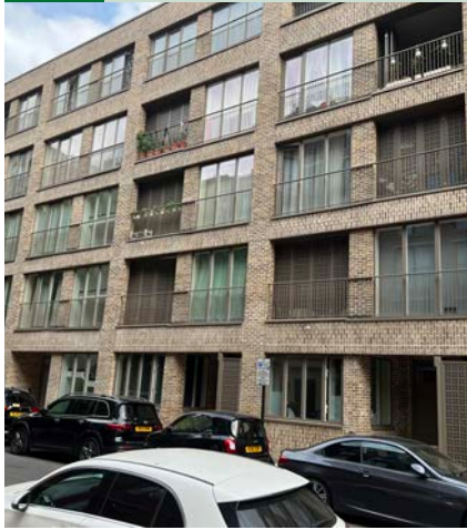
185 Recessed balconies are often more useful for residents, and can have openable glazing to turn them into winter gardens, or as here, metal perforated screens for shade and privacy.
