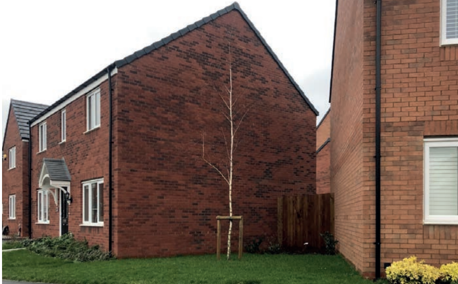
118 Blank gables are not a good way to turn a street corner.
