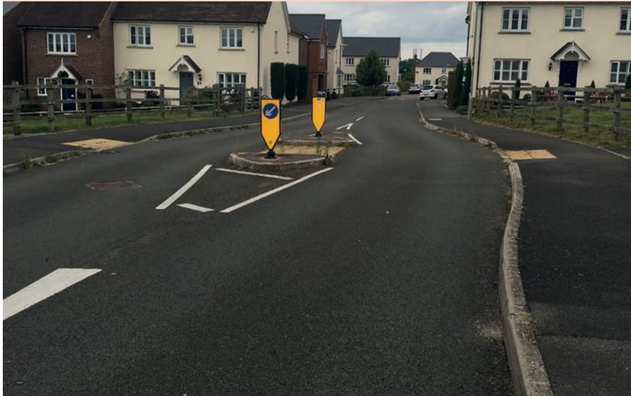
36 Features such as splitter islands are characteristic of higher speed roads than low speed streets.
