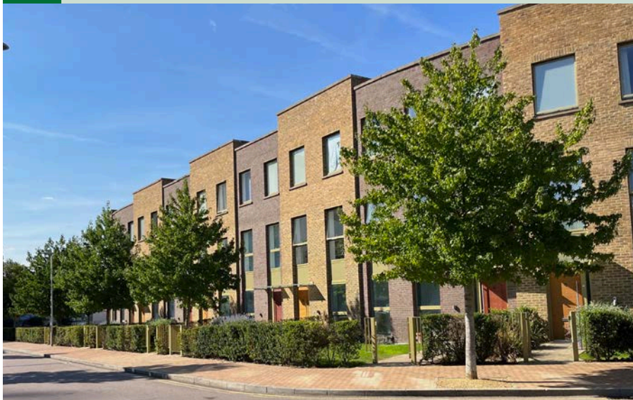
87 A mix of house types works best when form and materials create an obvious rhythm.
