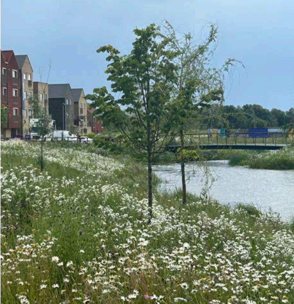
5 Attenuation basins created to capture water need to be designed as naturally as possible to maximise biodiversity and avoid unattractive, heavily engineered features.
