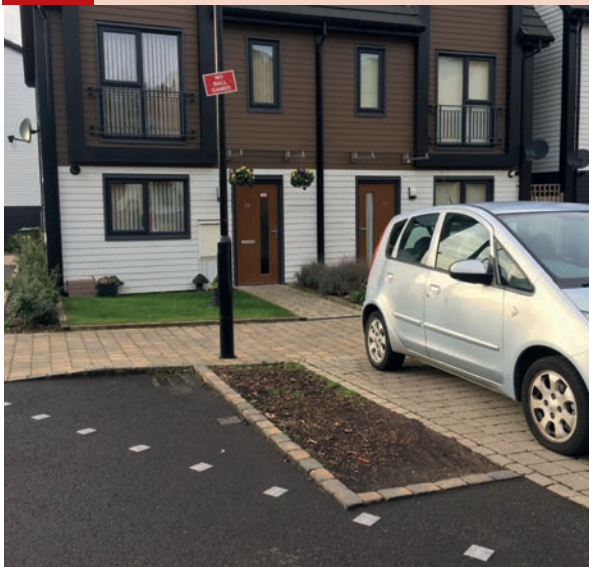
202 Landscaping between car parking spaces need some vertical protection to help establish planting.
