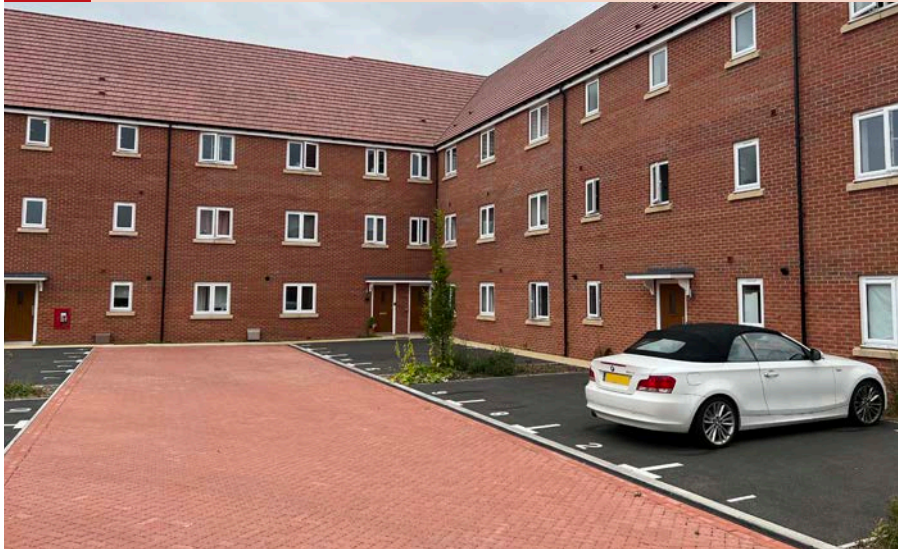
162 Apartments should not be exposed directly to the headlamps and exhausts of cars. A threshold needs to be created with either hard or soft landscaping to offer residents a good quality of life.
