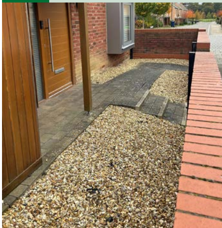
195 Where a house type is wide enough, a ramp provided laterally can supplement steps up to the front door from the pavement edge. Each of the two routes to this front door have their own street access.
