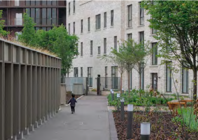
Image 35: Ryle Lane, Cambridge. Apartment external cycle storage pavilion.
