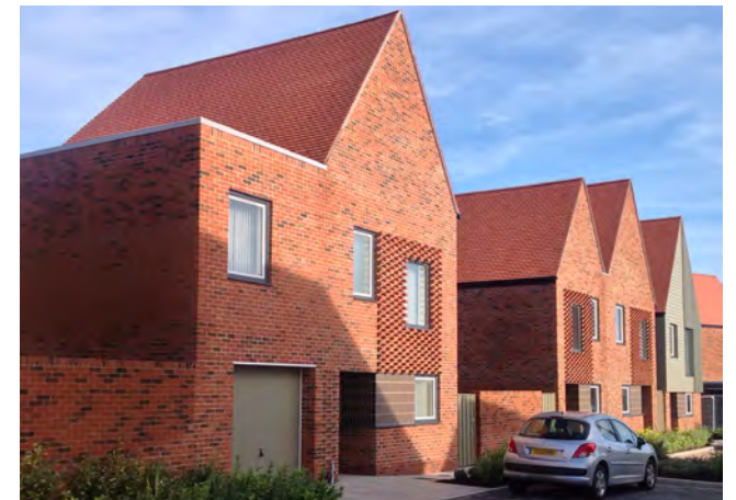
Image 27: Horsted, Chatham, Kent. House with integrated garage.
