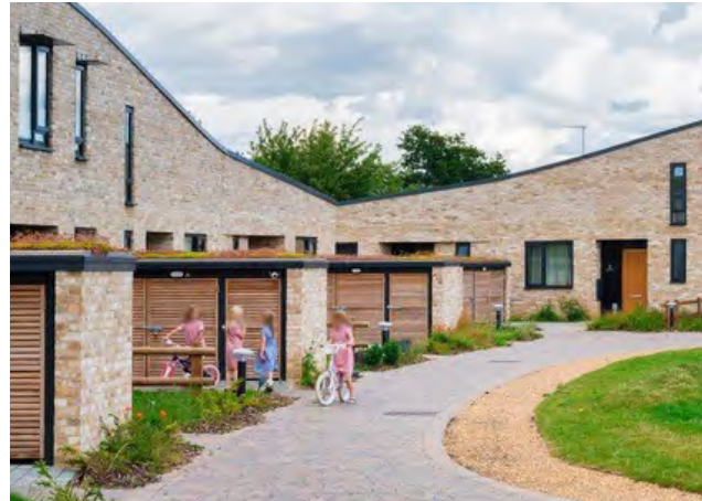
Image 30: More's Meadow. Bespoke timber store to the hard-standing of the houses.
