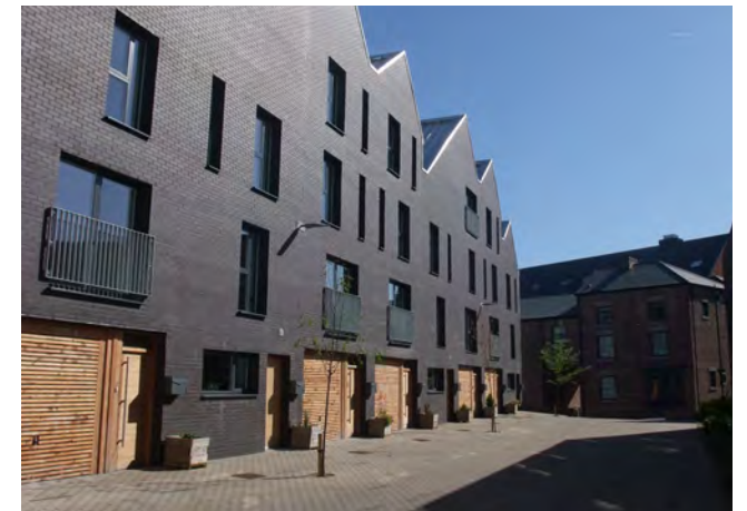
Image 28: Kelham Island, Sheffield. Block with integrated garages. Image 29: Accordia, Cambridge. House with integrated garages.
