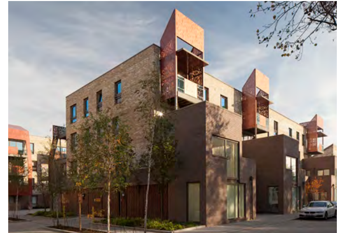
Image 58: Redwood Park, London. Undercroft car parking is screened with trees, planting and building projections.
