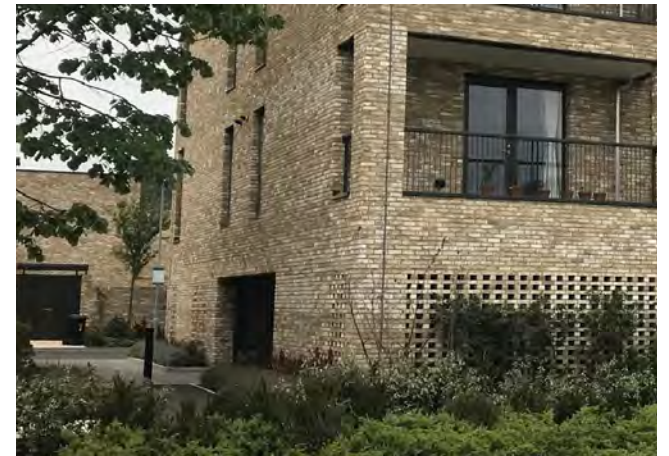
Image 59: Great Kneighton, Cambridge. Quality planting and feature brickwork screening the undercroft car parking.
