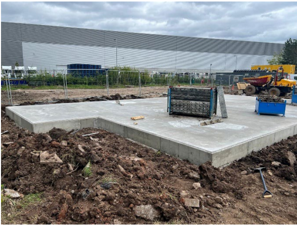
Figure 9. Foundations for chimney stack and pyrolysis kiln and thermal oxidiser
