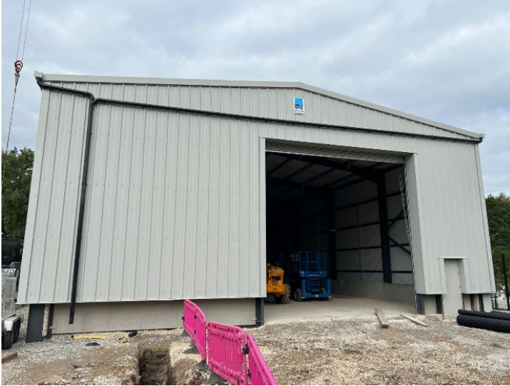
Figure 10. Erection of the fuel store building
