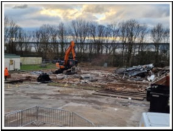
Figure 7. Demolition and clearing of site
