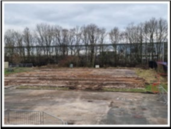
Figure 6. Demolition and clearing of site
