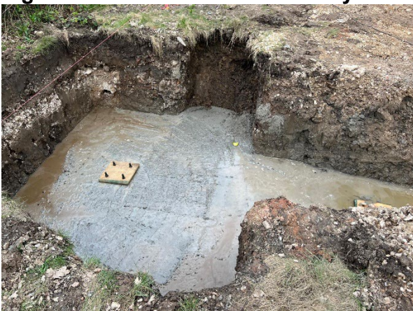
Figure 8. Foundations for chimney stack and pyrolysis kiln and thermal oxidiser
