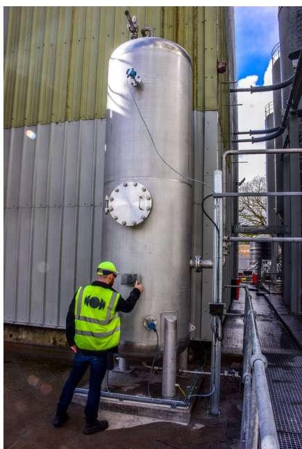
Figure 8: CO 2 buffer vessel and integration with OCO
