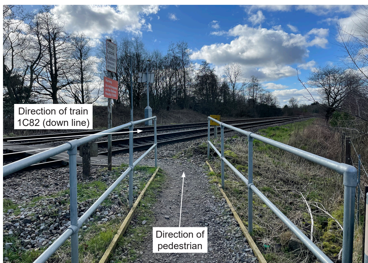
Figure 5: Approach to the crossing's north signage via the fenced corridor.
