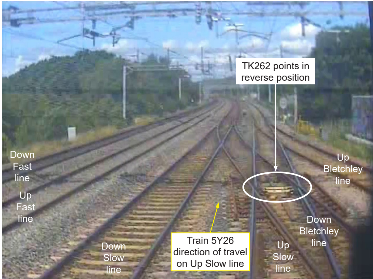
Figure 11: Forward-facing CCTV image from train 5Y26 showing the position of TK262 points (courtesy of West Midlands Trains with RAIB annotations).
