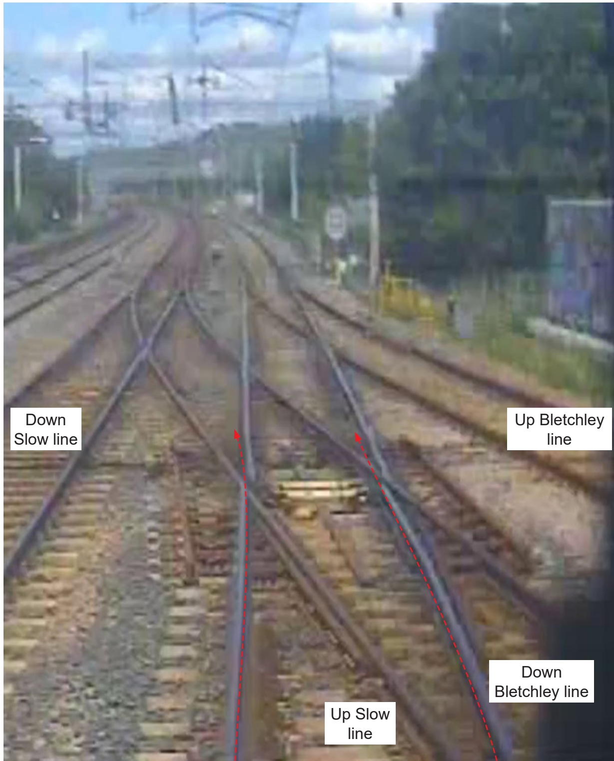
Figure 17: Path taken by the leading wheelset of train 5Y26 after approaching on the Up Slow line and then travelling through TK262A points and over TK262B points in their reverse position (courtesy of West Midlands Trains with RAIB annotations).
