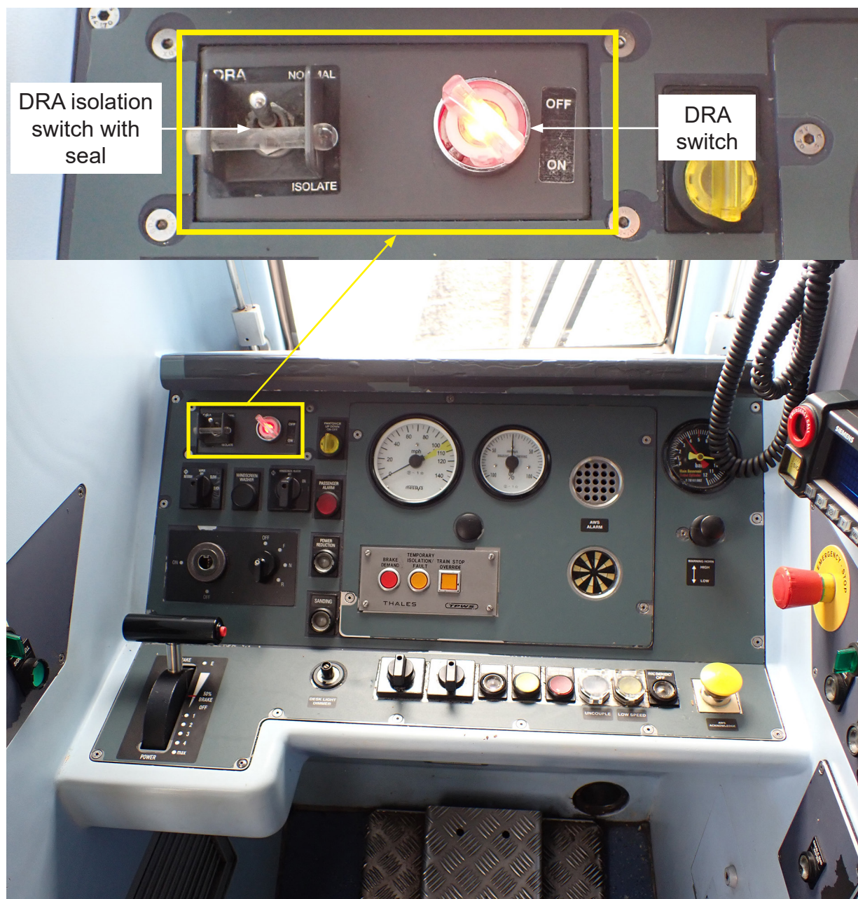
Figure 18: The DRA switch in the cab of a class 350 unit.
