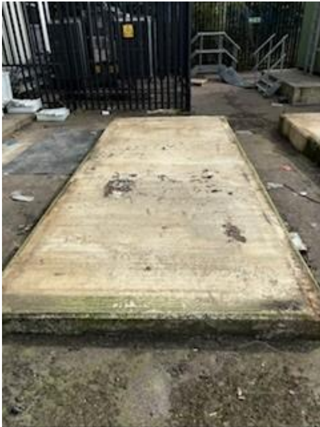
Photo C.5: Bulk Diesel Tank Concrete Base After Removal
