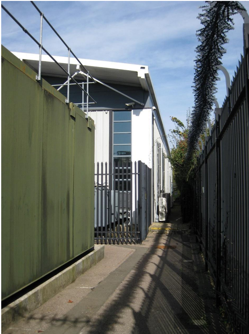
Photo C.3: Bulk Diesel Tank – rear view
