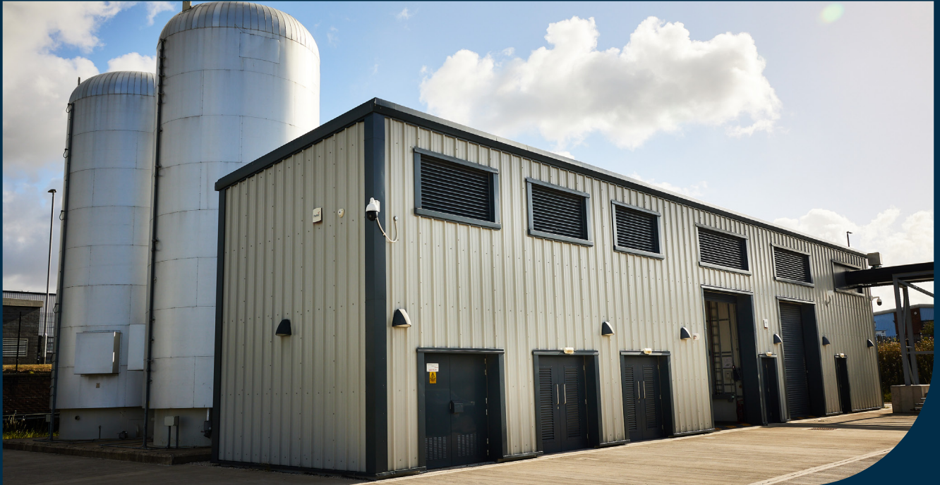
Energy Centre, Leeds. Courtesy of Vital Energi.
