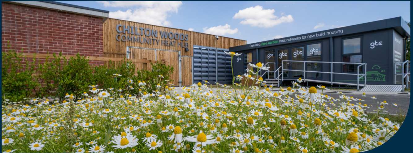
Chilton Woods Community Heat Hub.
