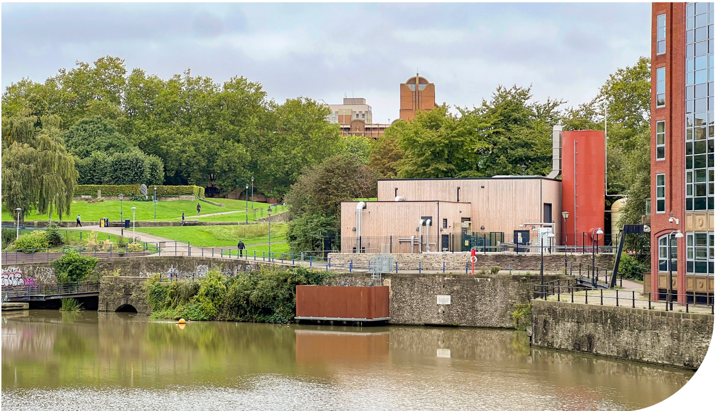
Castle Park Energy Centre water source heat pump.
