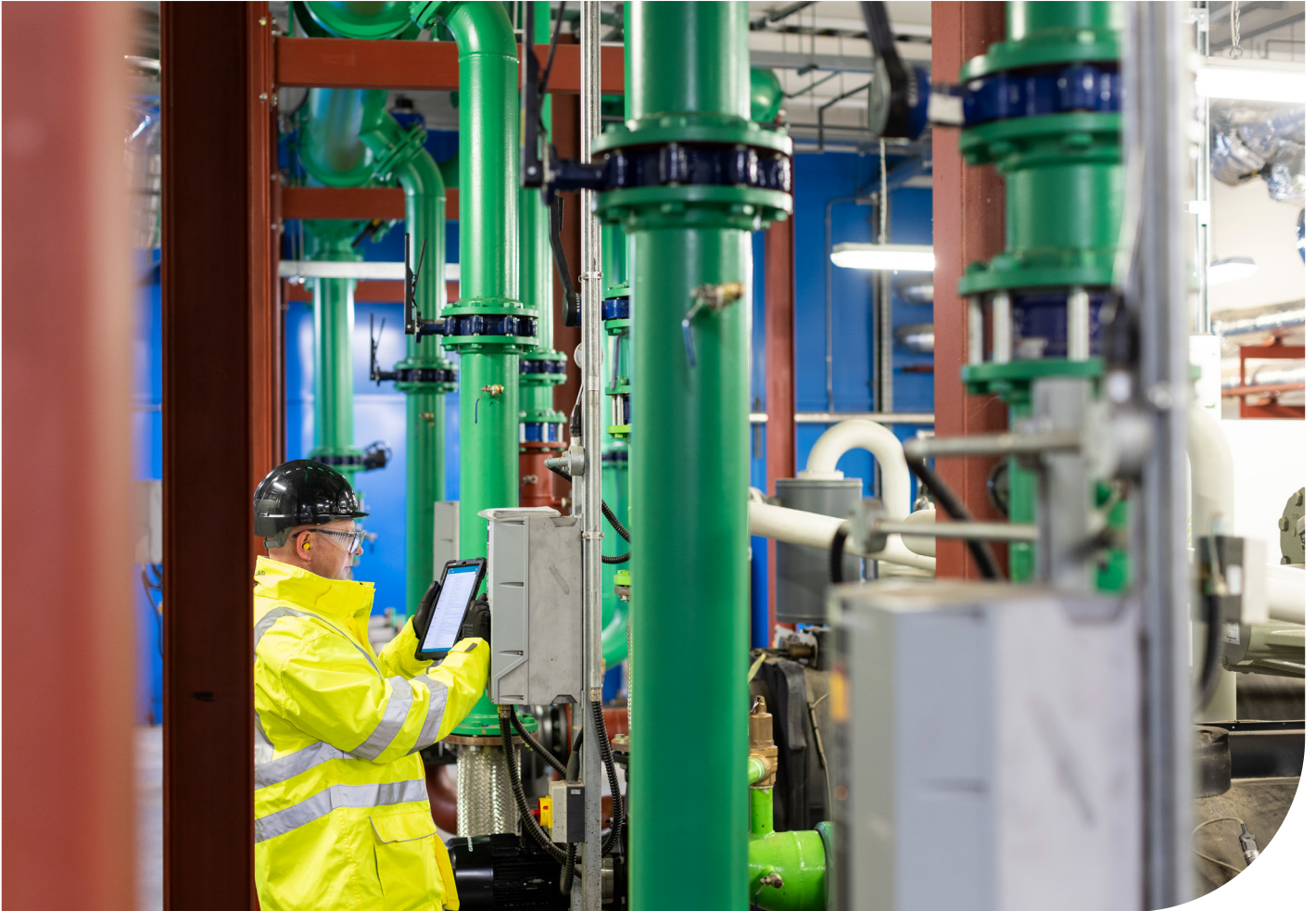
Credit: Birmingham heat network, Bring Energy / Simon Jarratt
