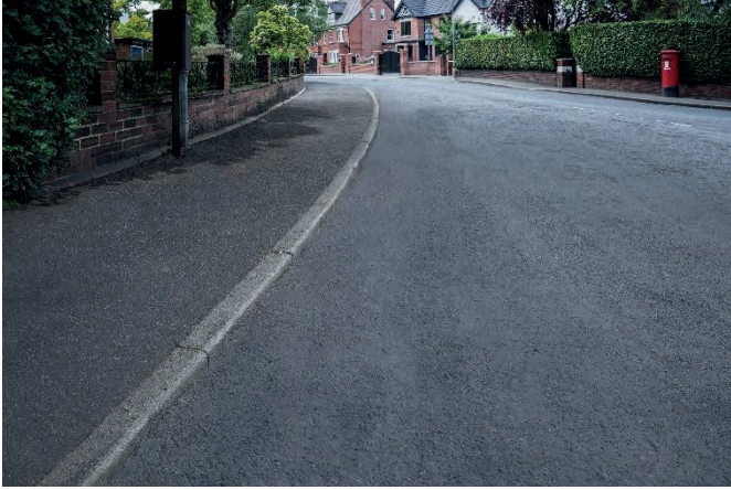
This image shows an urban road with no detritus. This means it is a grade A standard.
