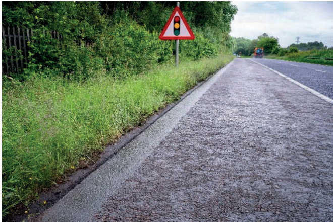
This image shows a major road with no detritus. This means it is a grade A standard.
