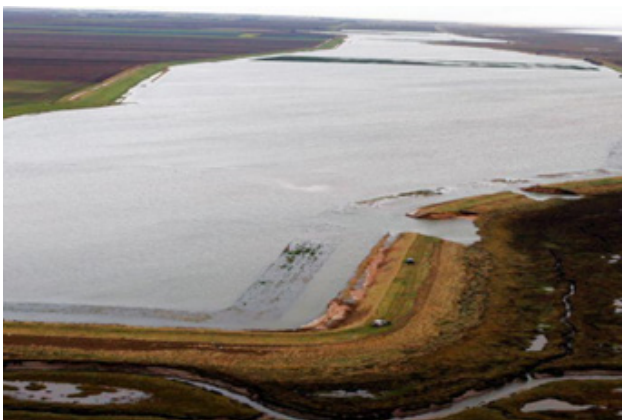
Tidal flooding of agricultural land near Wrangle in December 2013 © Environment Agency
