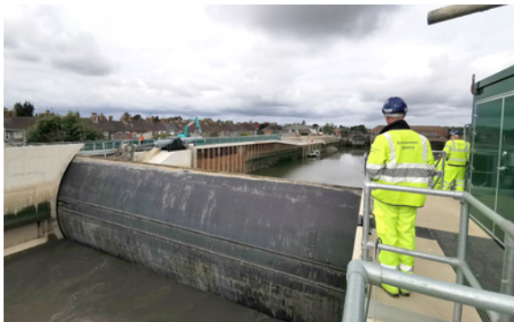
The Boston Barrier © Environment Agency
