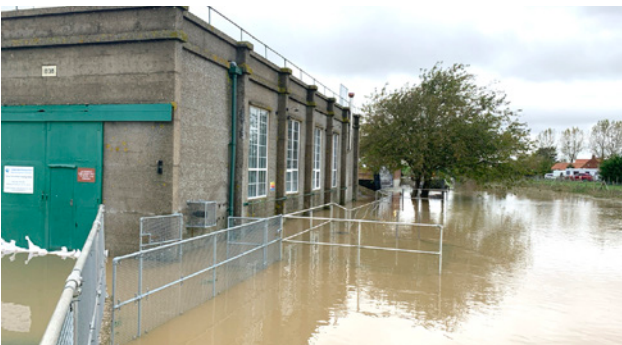
Overtopping of the Wainfleet Relief Channel in October 2023 threatened the operability of Thorpe Culvert Pumping Station © Environment Agency
