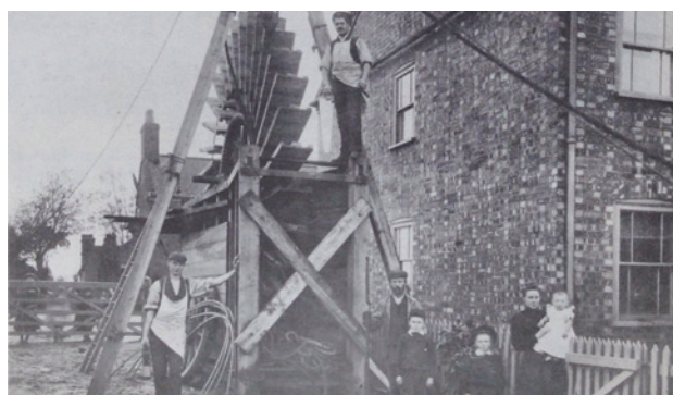
Horse-powered scoop wheel in Bourne South Fen, 1904 © Heritage South Holland.
