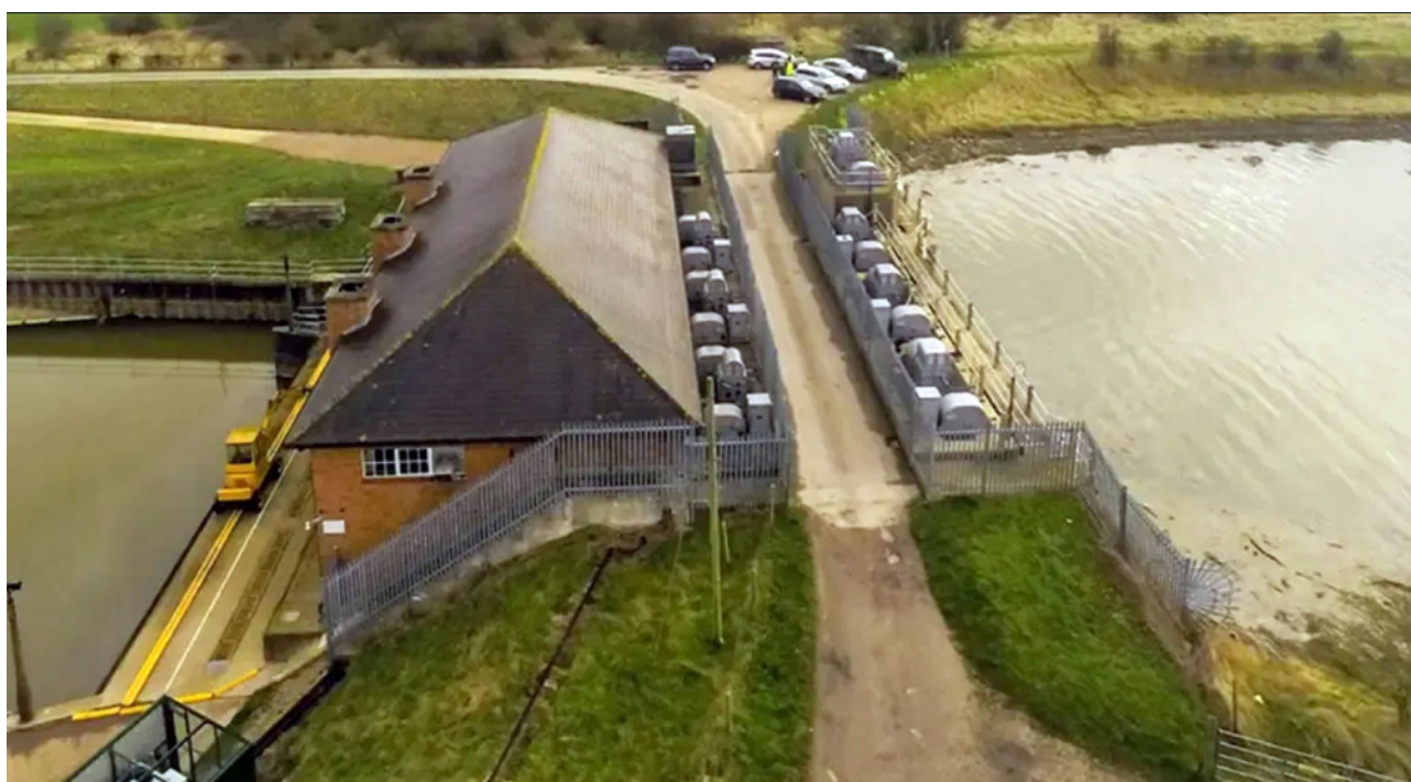
Hobhole Diesel Pumping Station, showing the difference in water level between the Hobhole Drain (left) and the Boston Haven (right) into which water must be pumped © Witham Fourth District IDB.
