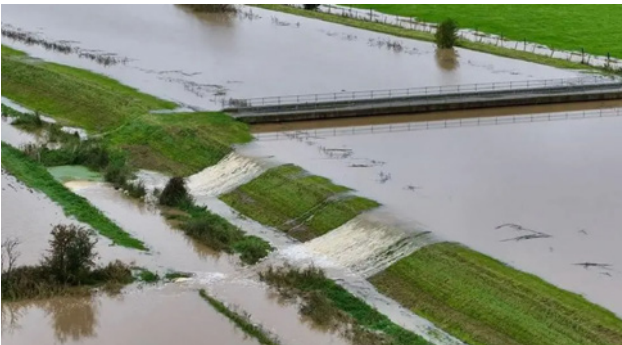
Overtopping of the Wainfleet Relief Channel during Storm Babet in October 2023 © BBC 2023
