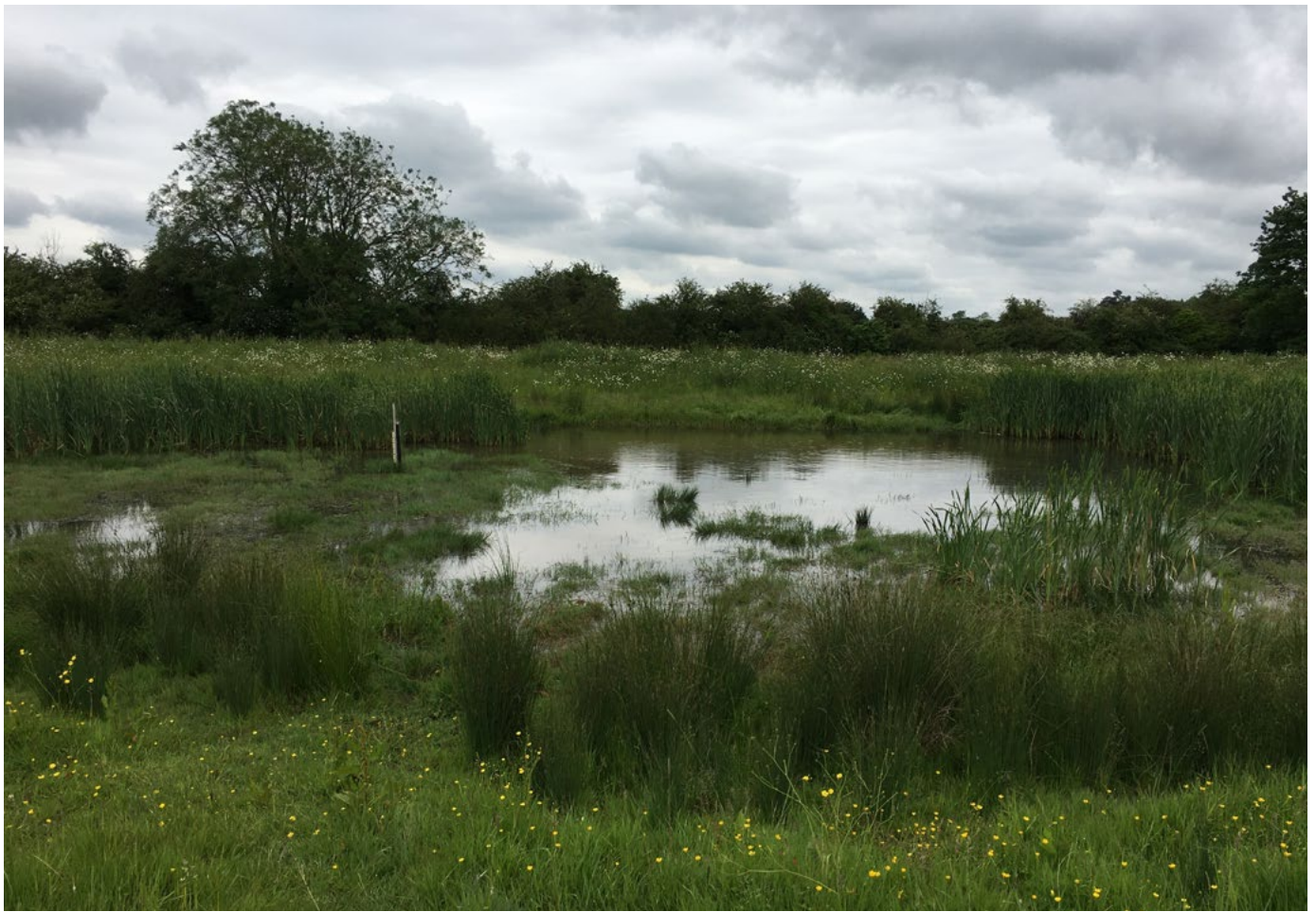
Run-off attenuation ponds in the Evenlode catchment designed to slow the flow of water through the landscape and retain nutrients.
