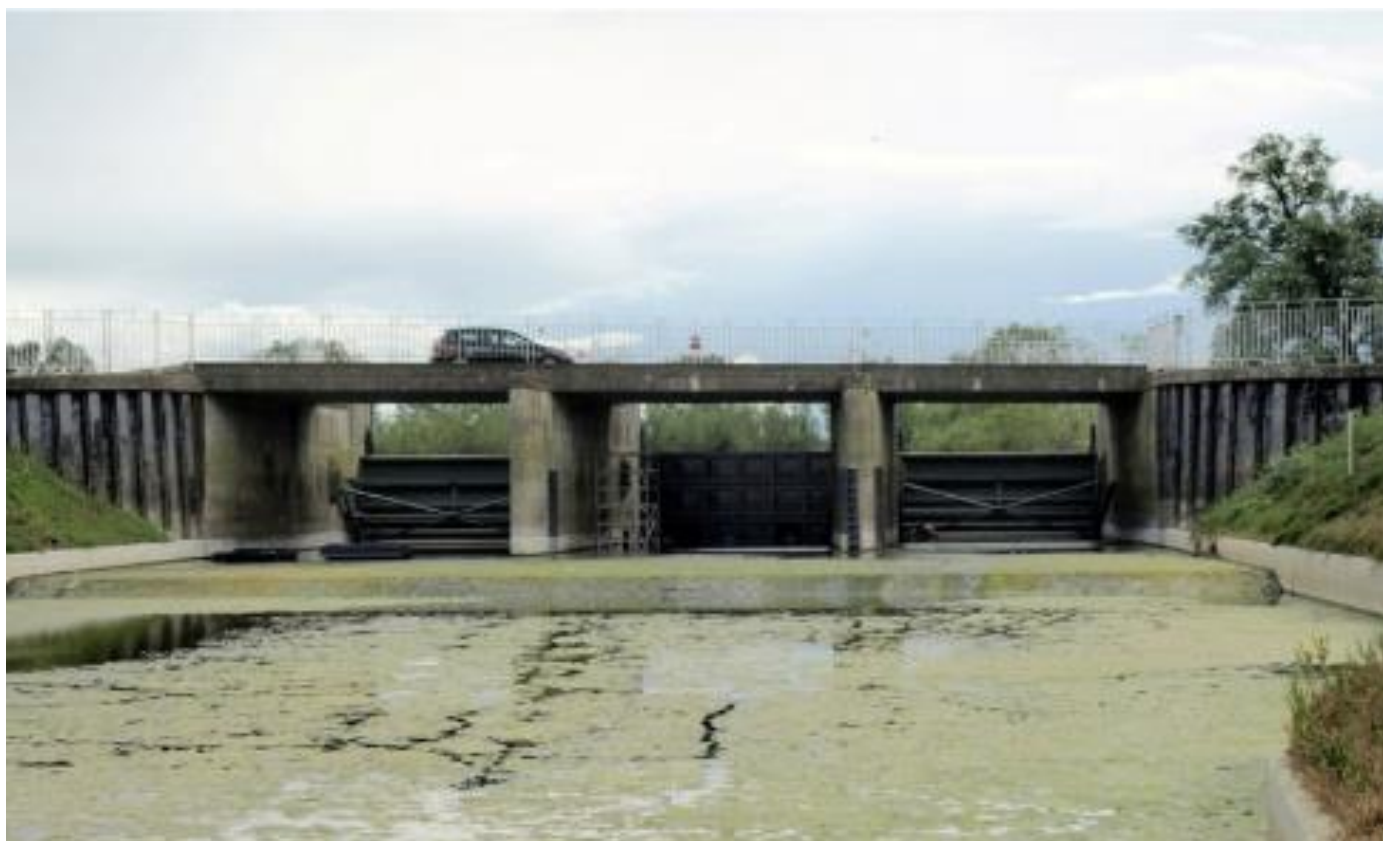
Figure 8: Earith Sluice looking South (upstream) © ousewashes.info
