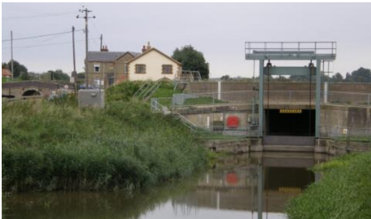
Figure 16: Old Bedford Sluice looking North-East (downstream) 16
