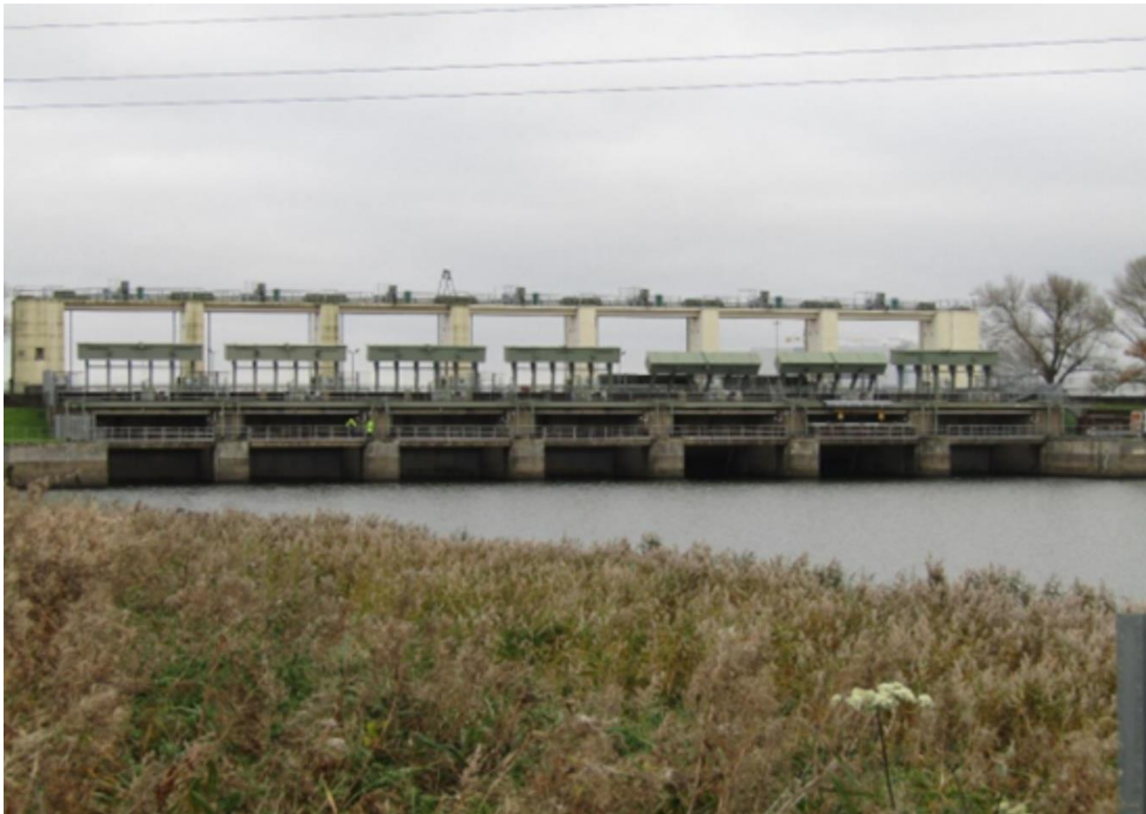
Figure 17: Tail Sluice looking North (downstream) (Environment Agency)
