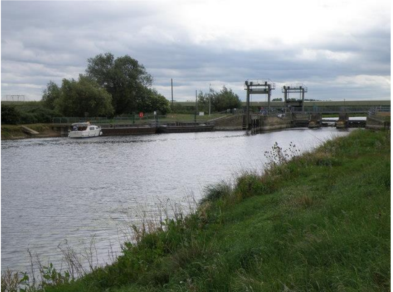
Figure 7: Brownhill Stauch Sluice looking South (upstream) © Michael Trolove and licensed for re-use under the Creative Commons Licence.
