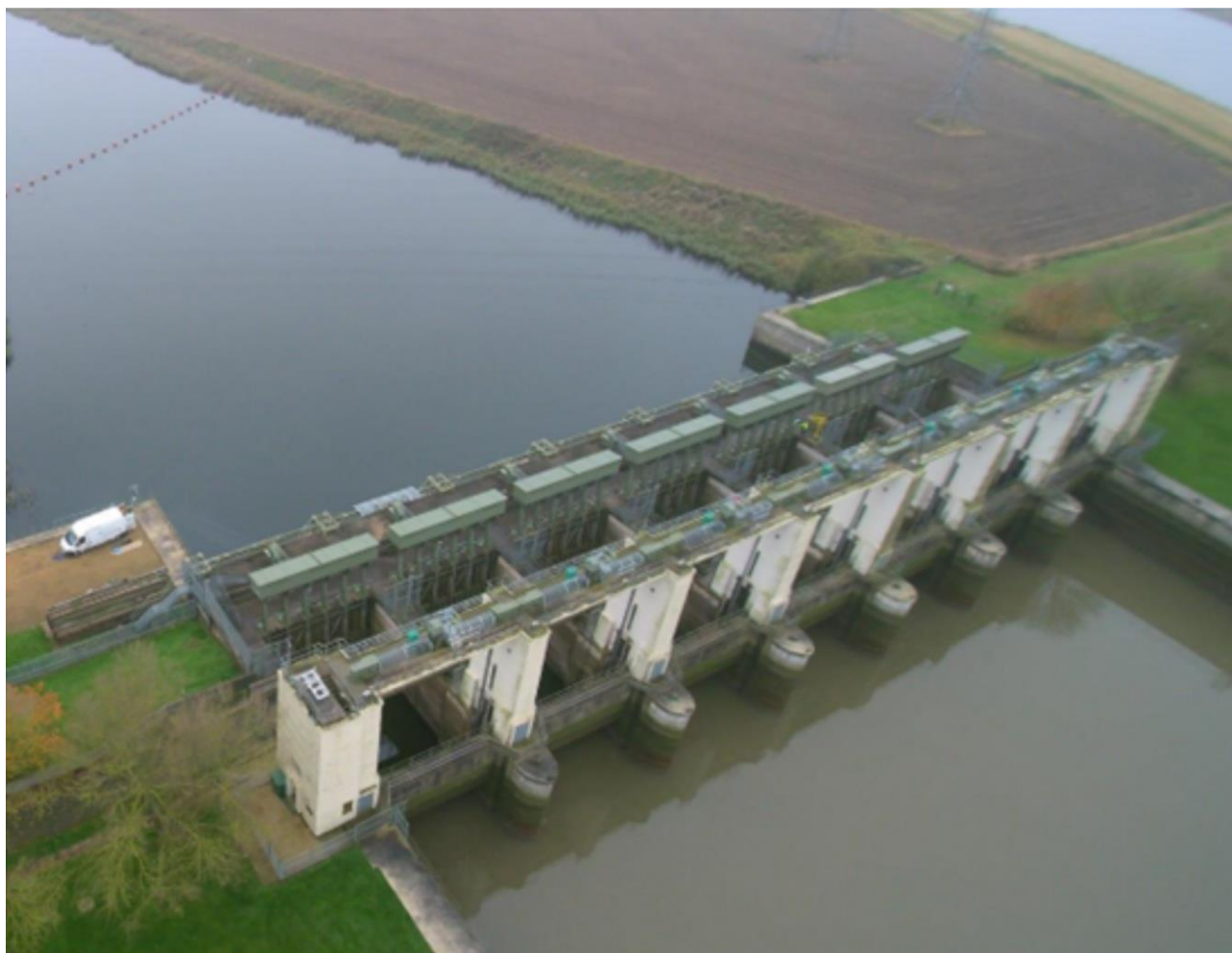
Figure 18: Tail Sluice looking South (upstream) (Environment Agency)
