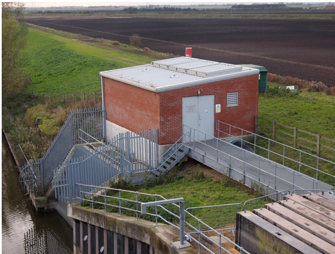
Figure 20: Welmore Lake Pumping Station looking West (2017) © ousewashes.info
