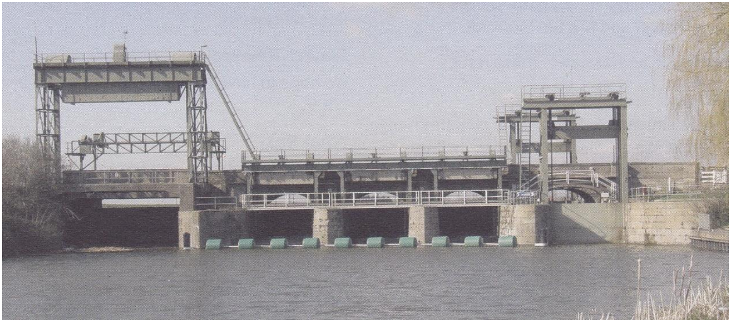
Figure 12: Denver Sluice looking North (downstream) 9
