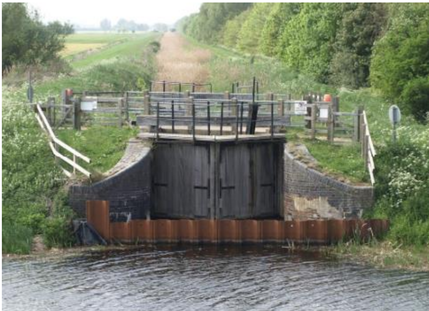
Figure 9: Welches Dam Lock looking West (upstream) (April 2011) © ousewashes.info
