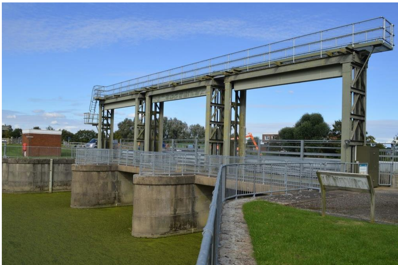
Figure 14: Impounding Sluice looking North (downstream) 13
