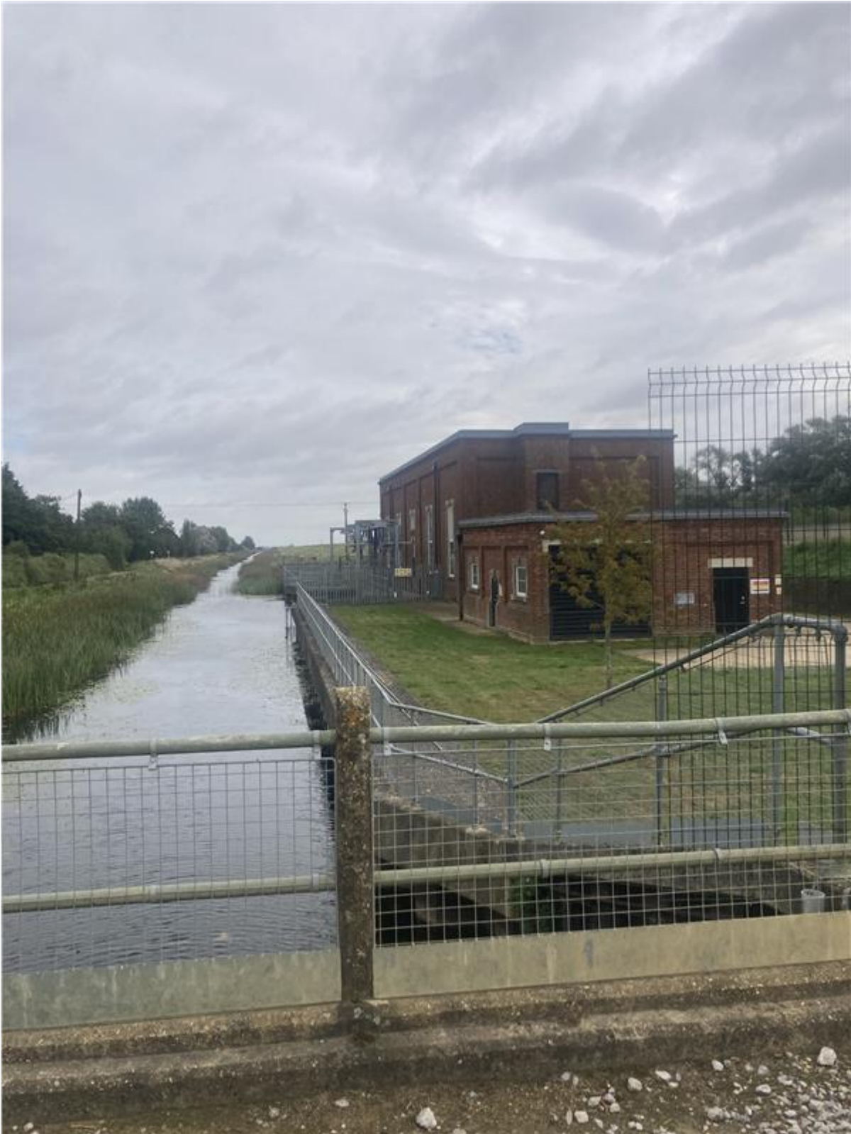
Figure 19: Welches Dam Pumping Station looking North-East (downstream) (© Arup 2024).
