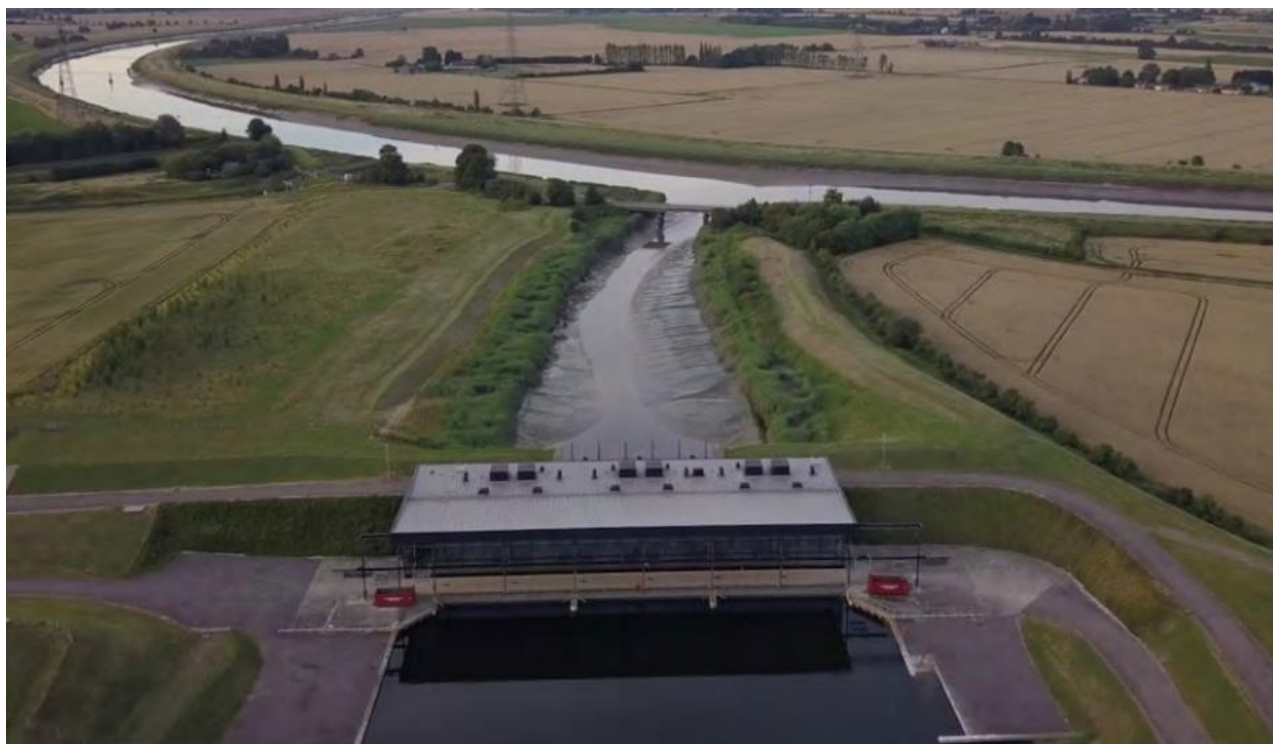
Figure 21: St Germans Pumping Station looking North (upstream) © Environment Agency
