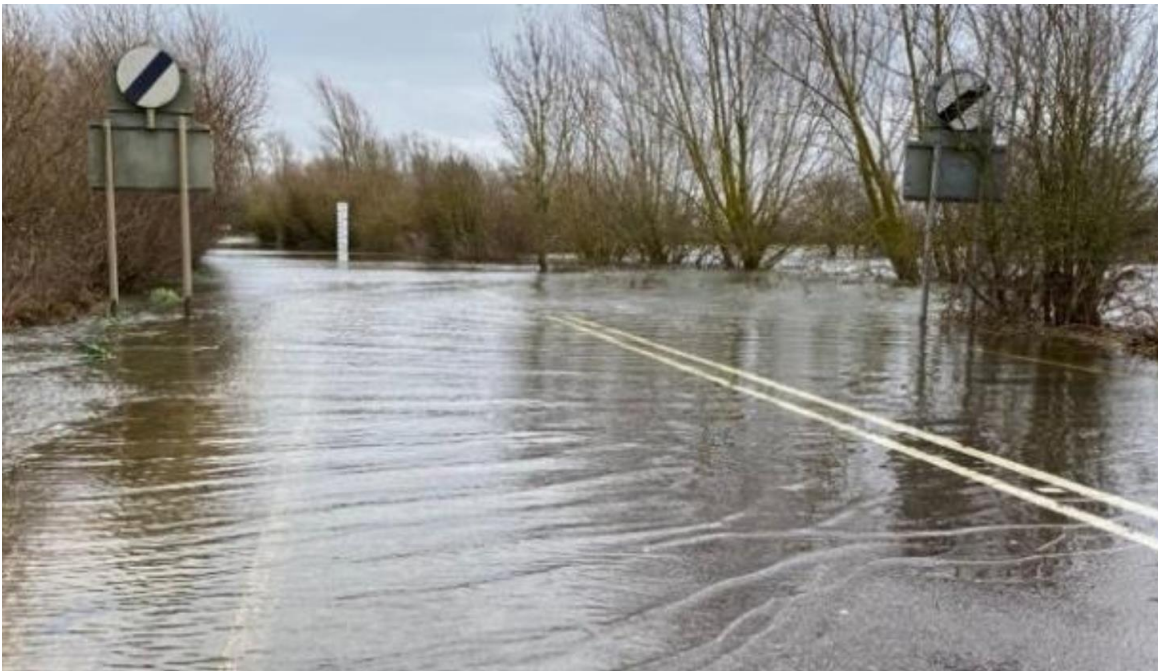
Figure 41: Flooded A1101 March 2023 62
