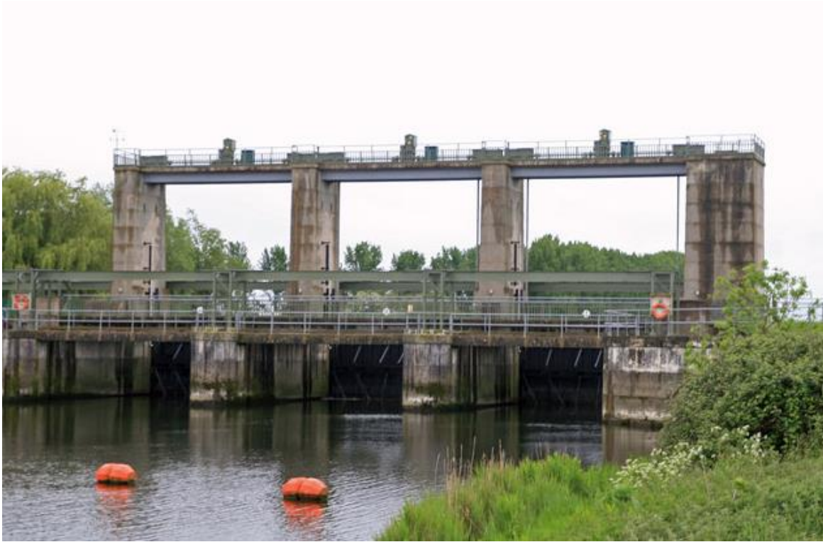
Figure 13: A.G Wright Sluice looking South (upstream) 11
