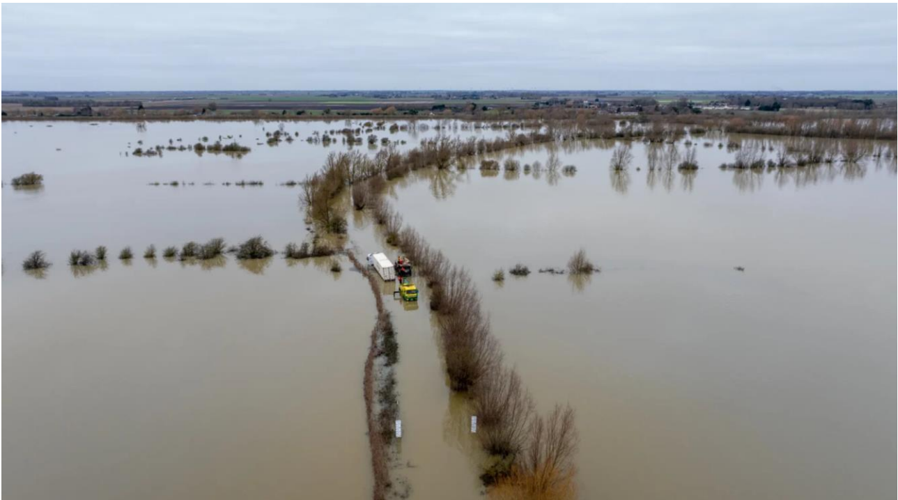
Figure 42: Flooded A1101 January 2024 63
