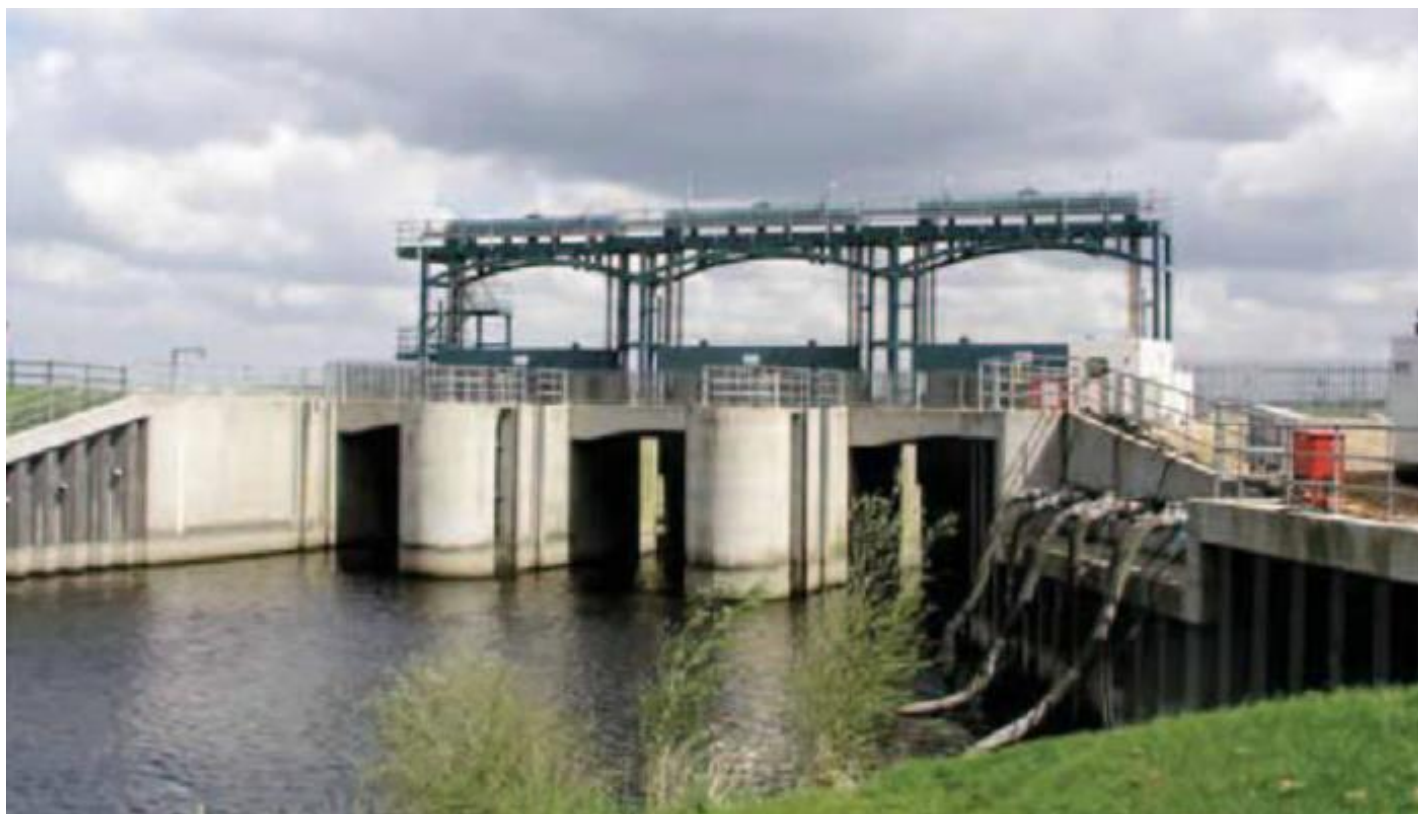
Figure 10: Welmore Lake Sluice looking North-East (downstream) © ousewashes.info
