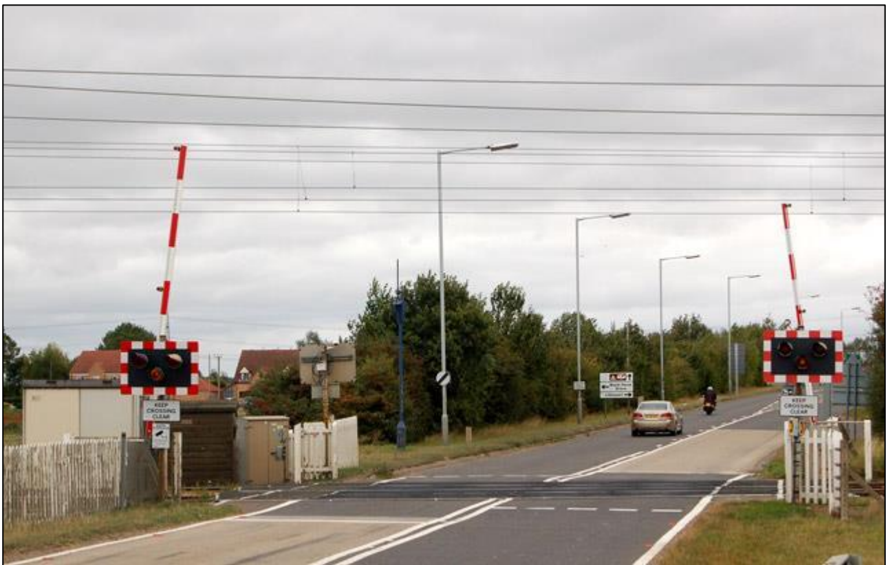
Figure 15: Littleport bypass level crossing (A10)
