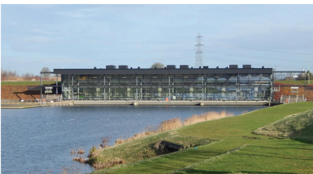
St. German's Pumping Station © Fascinating Fens.
