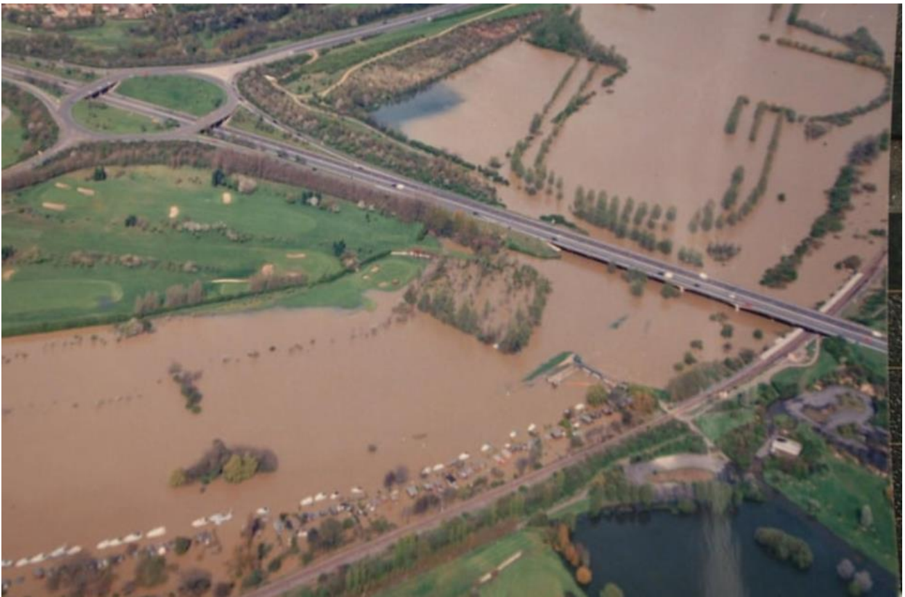
Figure 15: 1998 flooding at Orton Mere
