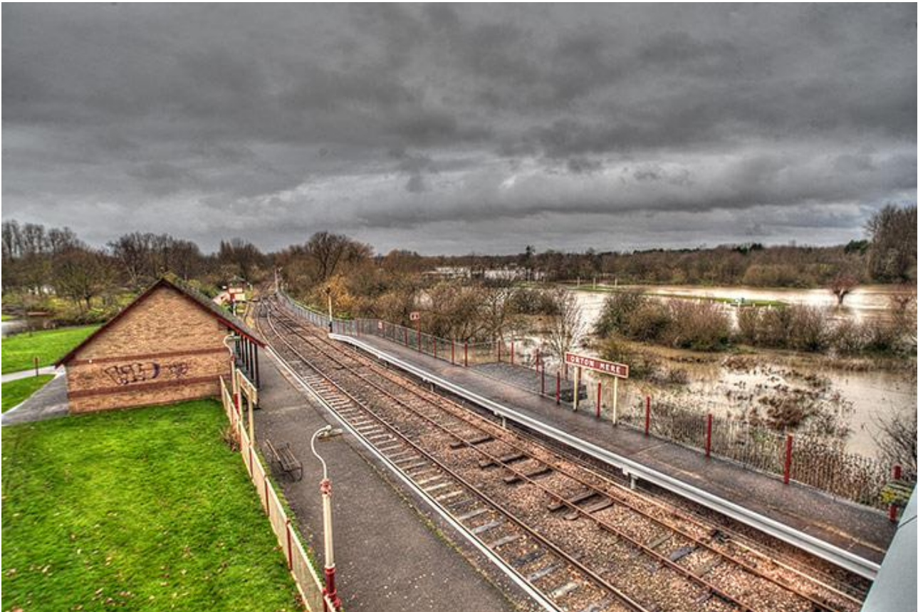
Figure 16: River Nene flooding at Orton Mere 7
