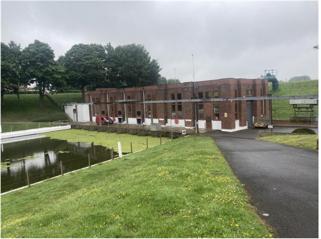
Figure 5: Tydd Pumping Station (© Copyright Arup 2024)
