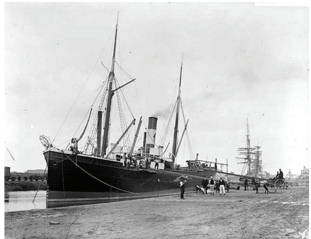
Photograph of Wisbech Port in 1899 © by permission of Historic England Archive
