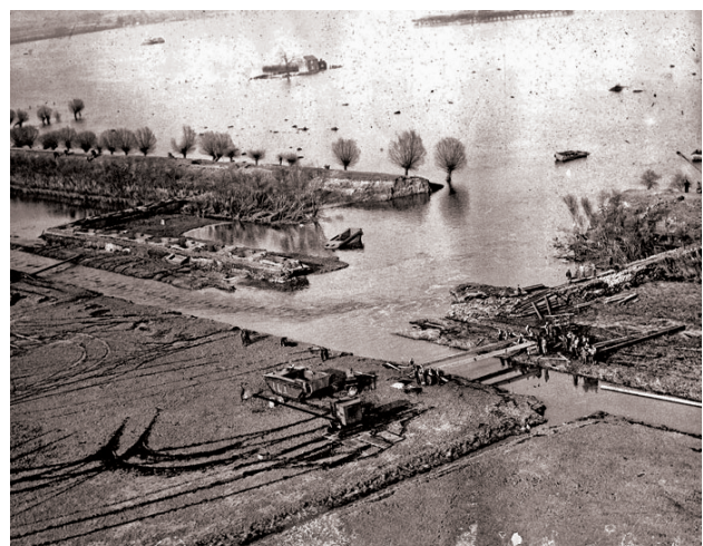
Photograph of the 1947 flooding of the North Level District caused by heavy rain and a breach in the Crowland and Cowbit Washes © Peterborough Images Archive, 2018
