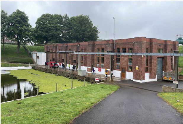
Tydd Pumping Station © Arup 2024.
