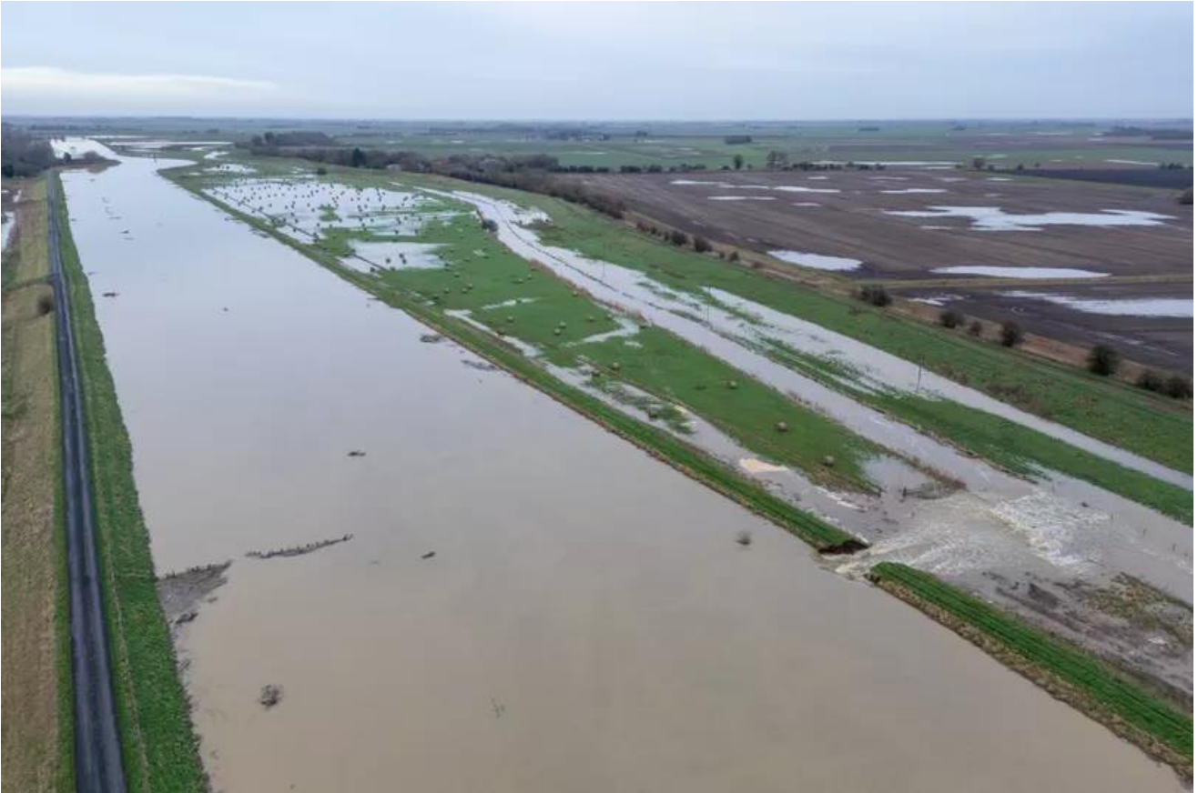
Figure 24: River Welland breach near Cowbit and Crowland © Lincolnshire Live
