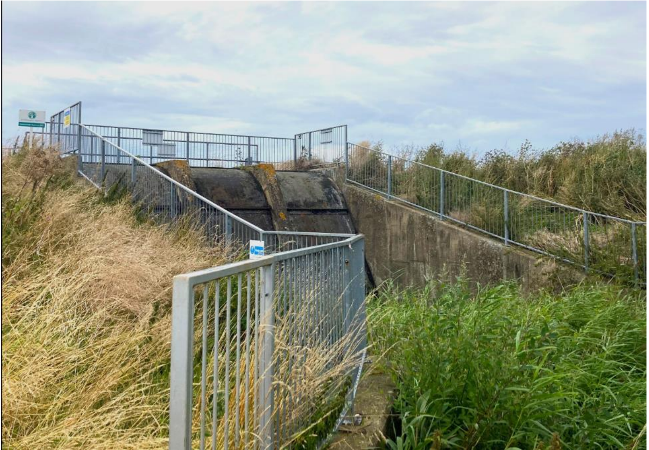
Figure 13: External view of the Newborough Siphon © Environment Agency
