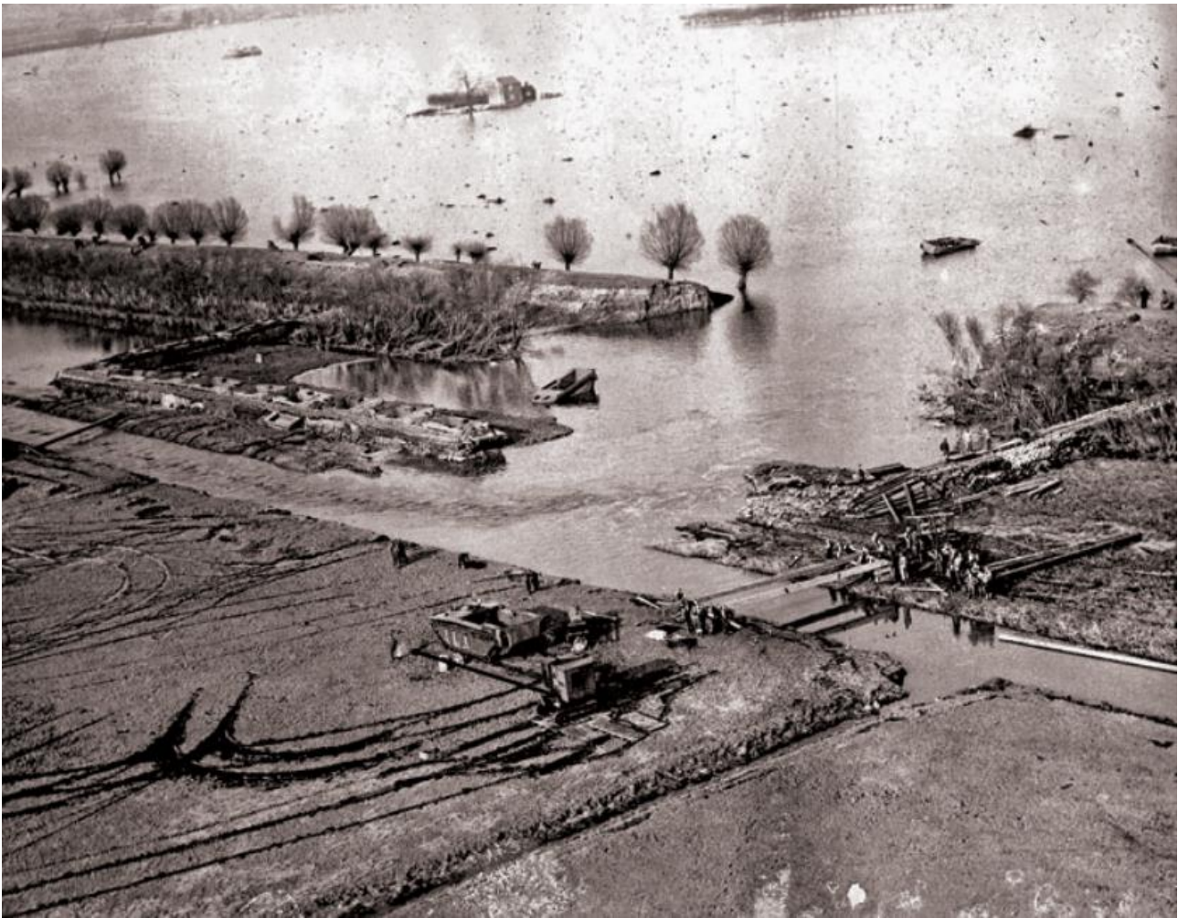
Figure 16: Historical photograph of the Barrier Bank breach following the flooding event of 1947 © Peterborough Images Archive
