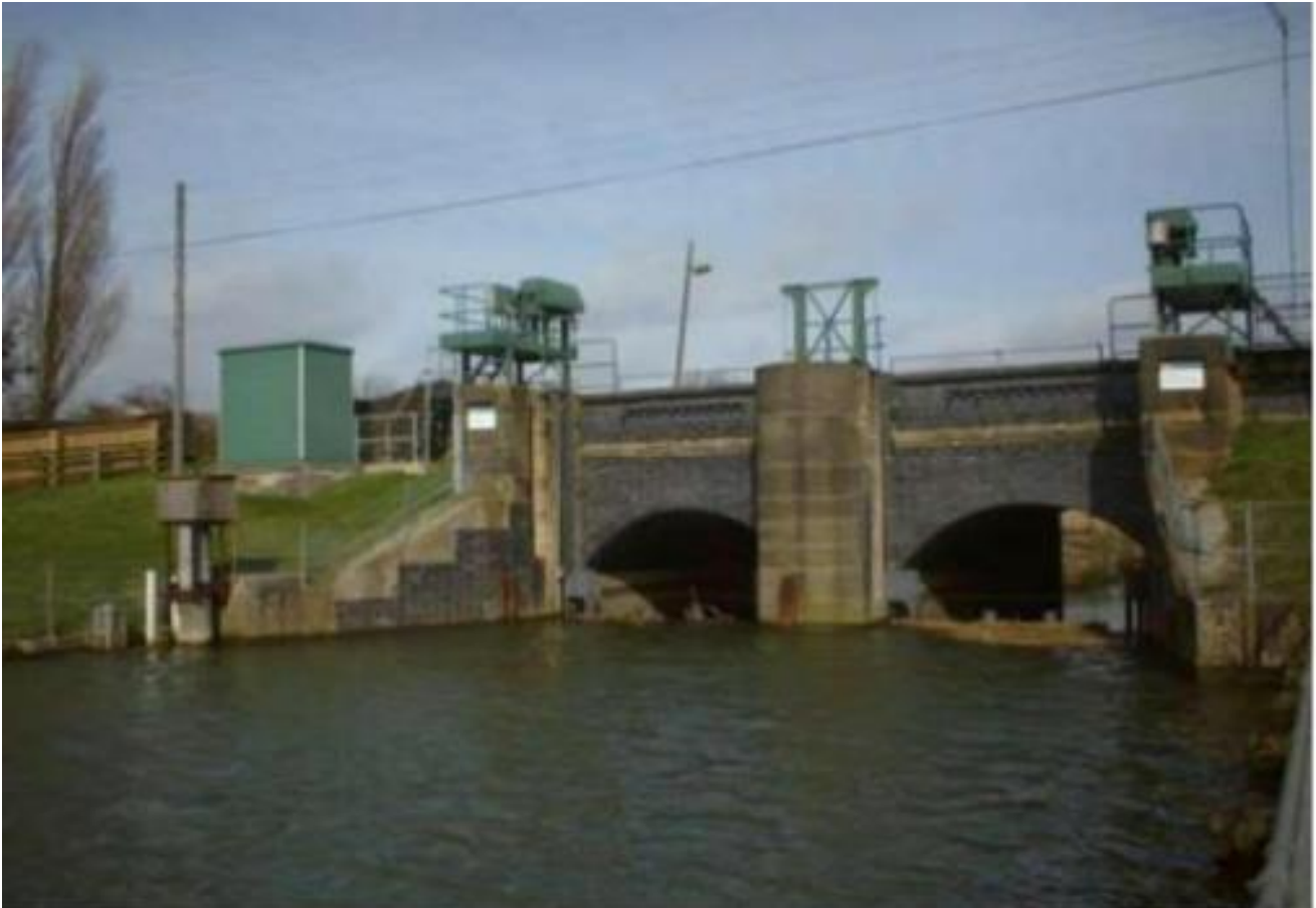
Figure 5: Upstream (reservoir) side of Surfleet Sluice © Environment Agency
