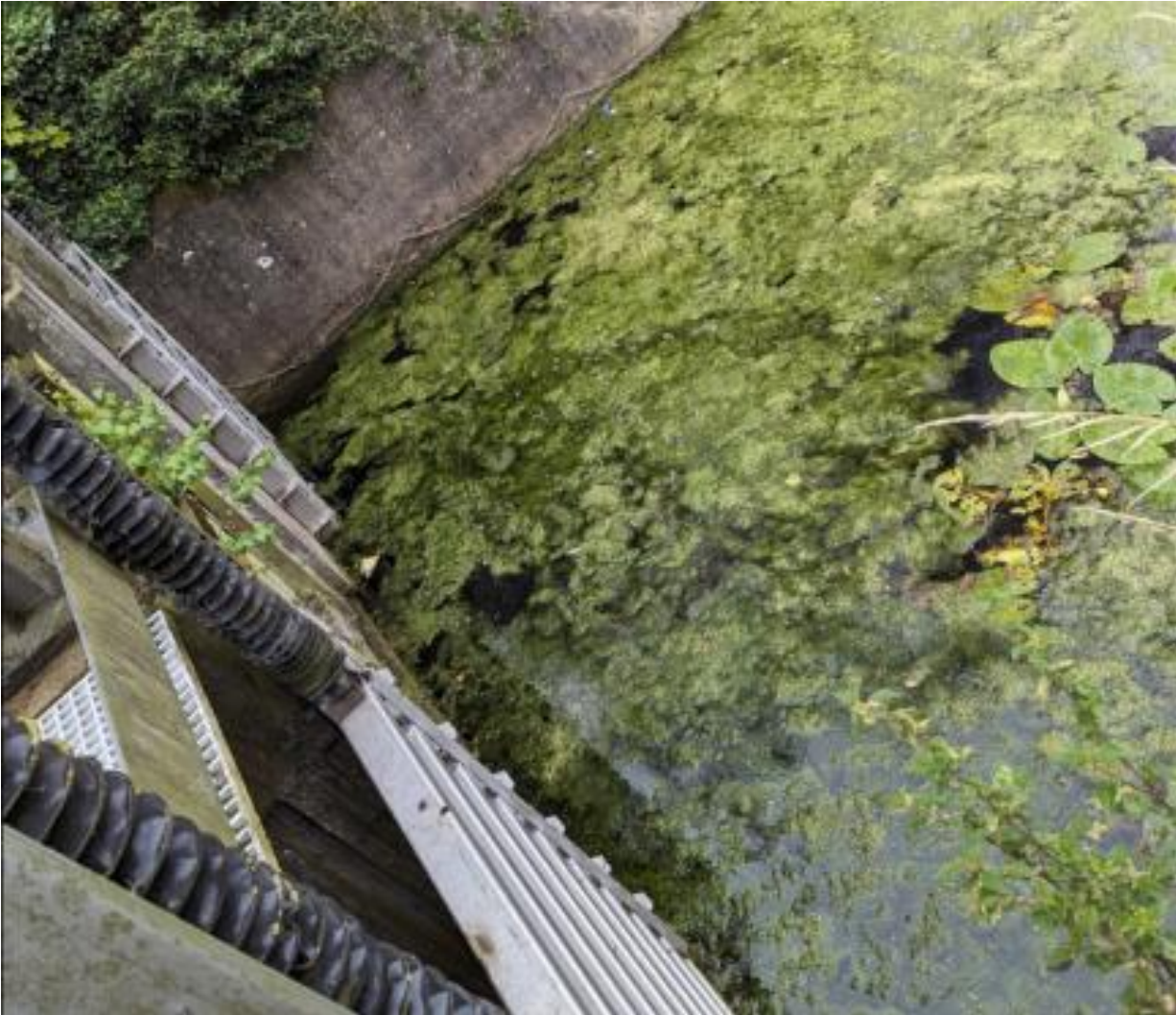
Figure 8: Locks Mill Sluice on Welland Side 3
