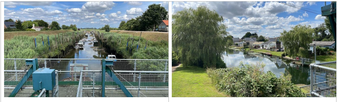
Figure 11: Photograph (left) of raised earthworks (tidal defences) at Surfleet Sluice (looking downstream) and Photograph (right) of Surfleet Reservoir. Houses built within the online storage area and within the raised defences (not seen, set back).
