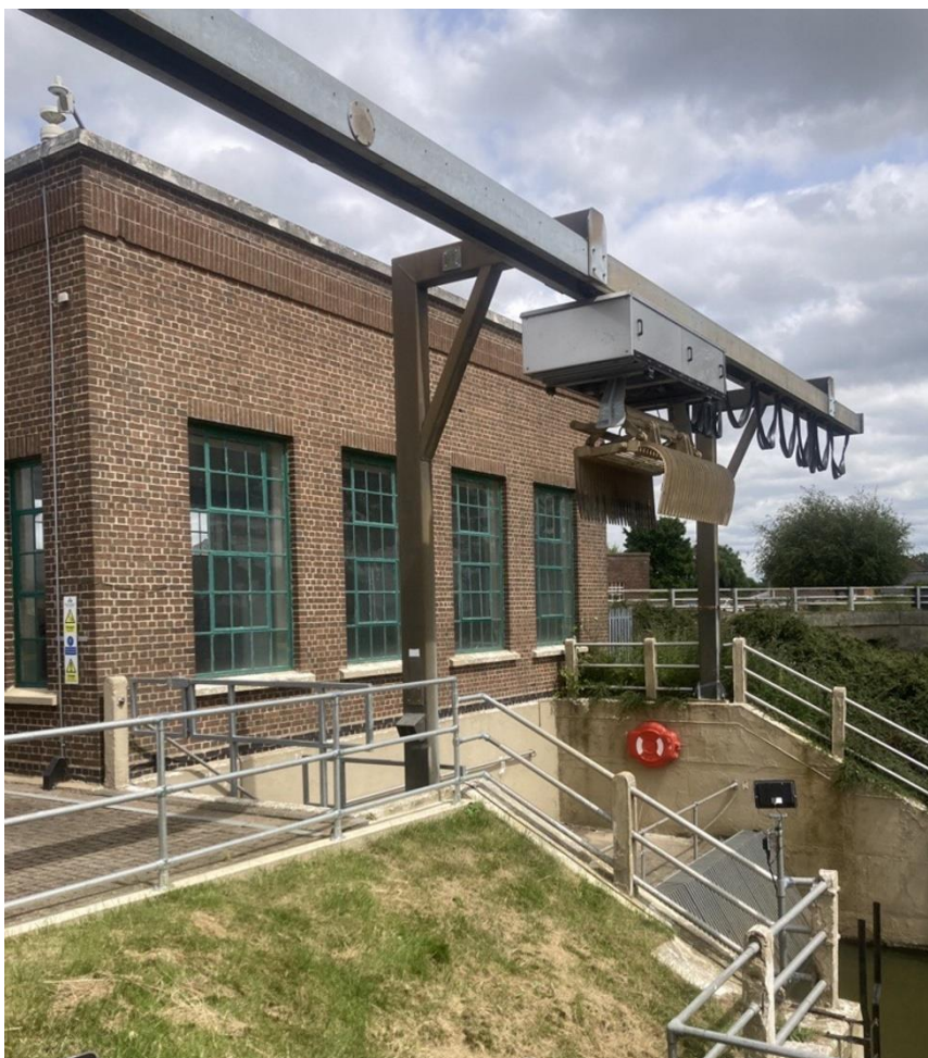
Figure 3: Deeping St Nicholas Pumping Station at Pode Hole
