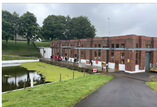
Tydd Pumping Station © Arup 2024.
