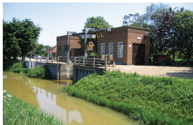
Bourne South Fen Pumping Station © Rodney Burton. Licensed for reuse under the Creative Commons Licence.
