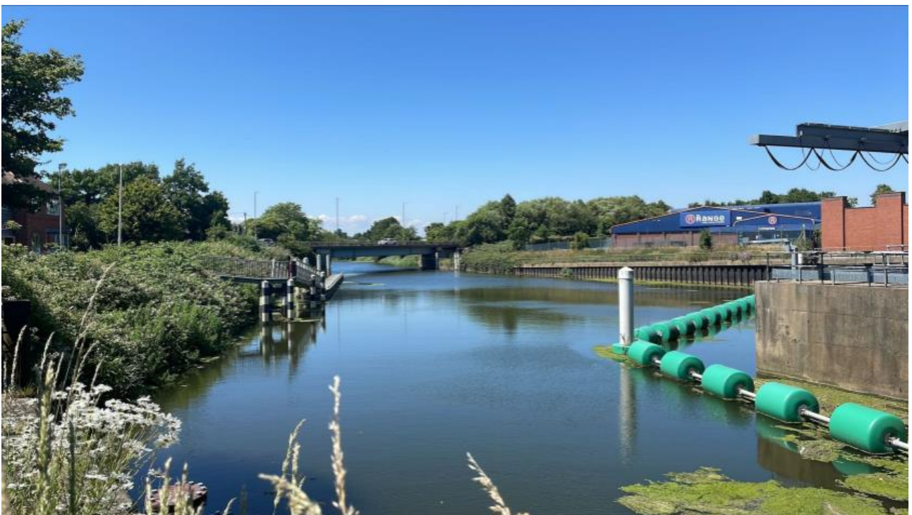
Figure 6: View from Black Sluice looking upstream © Arup
