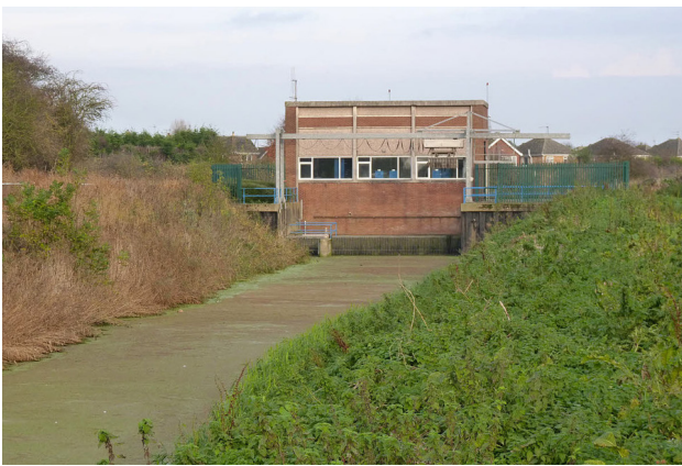
Chain Bridge Pumping Station © Alan Murray-Rust. Licensed for reuse under the Creative Commons Licence.
