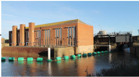
Black Sluice Pumping Station (now disused) © J.Hannan-Briggs. Licensed for reuse under the Creative Commons Licence.
