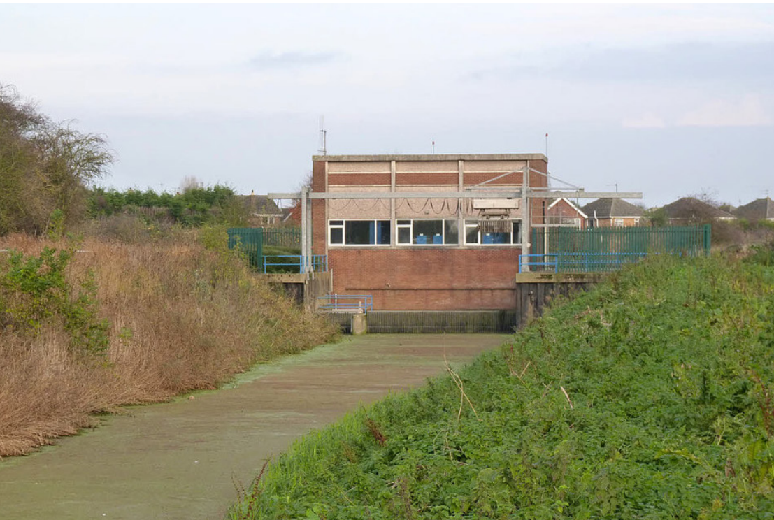
Chain Bridge Pumping Station is typical of the pumping stations built across the catchment in the 1960s © Black Sluice IDB
