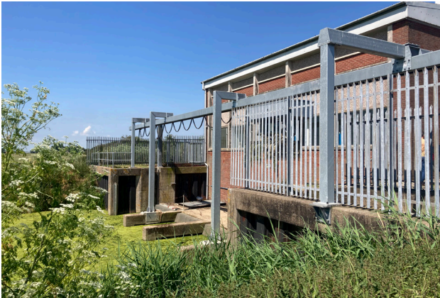
Swineshead Pumping Station © Arup 2024
