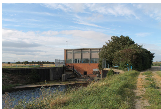
Black Hole Drove Pumping Station. © J.Hannan-Briggs. Licensed for reuse under the Creative Commons Licence.
