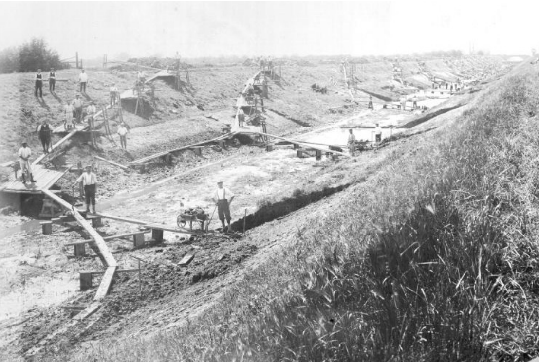
Drain cutting in the Black Sluice District © Black Sluice IDB
