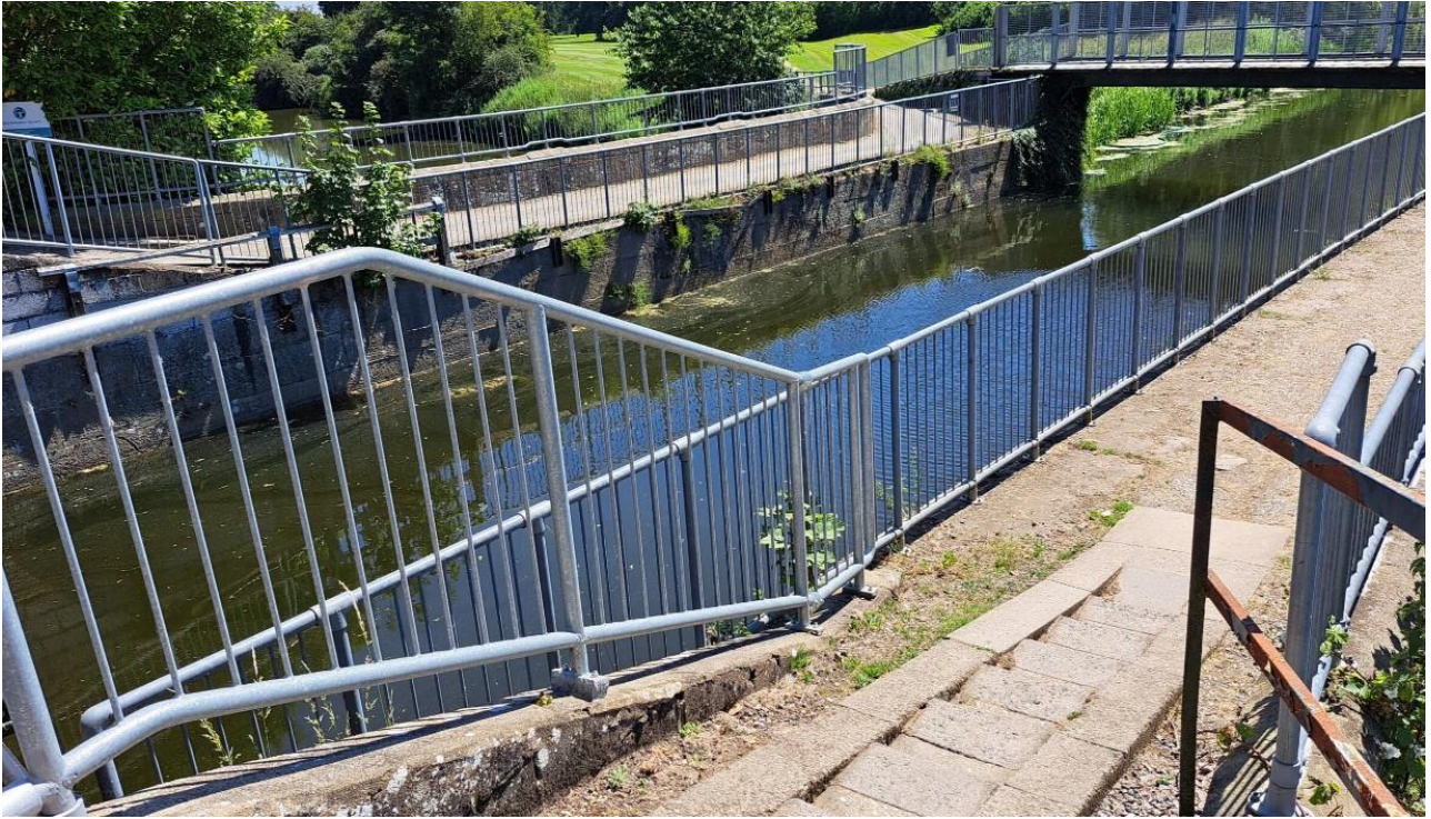
Figure 6: Stone Bridge Drain Aqueduct © Arup
