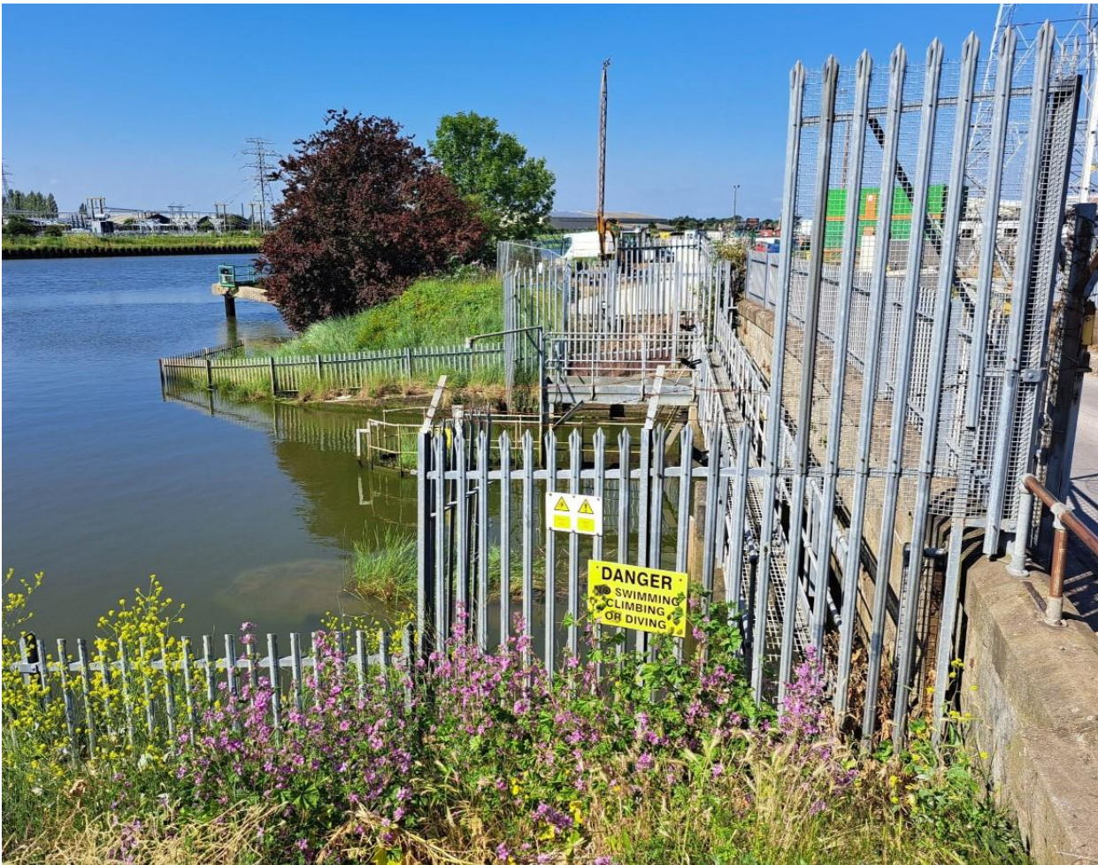
Figure 7: Maud Foster Sluice © Arup
