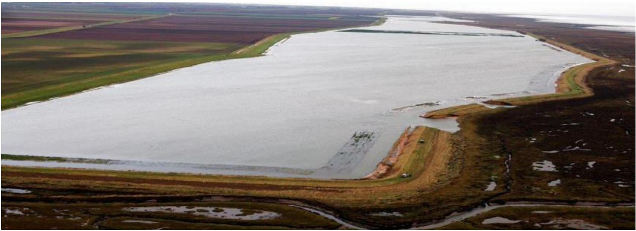
Figure 14: Image showing flooding due to breach at Wrangle © Environment Agency
