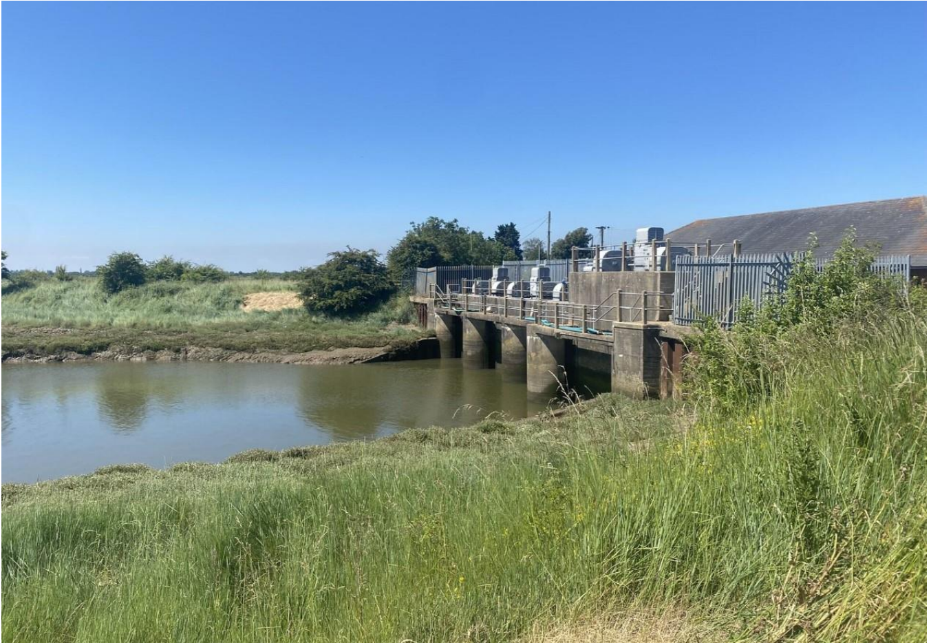
Figure 8: Hobhole Pumping Station © Arup
