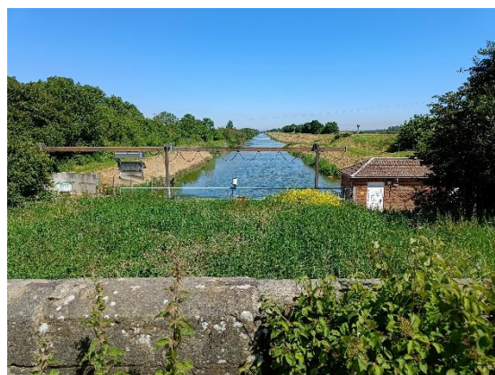
Figure 1: East and West Fens catchment (taken from Hobhole Pumping Station) © Hannah Smith
