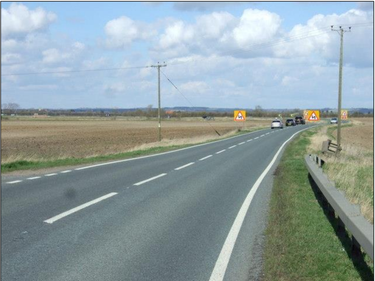
Figure 14: Main road A16
