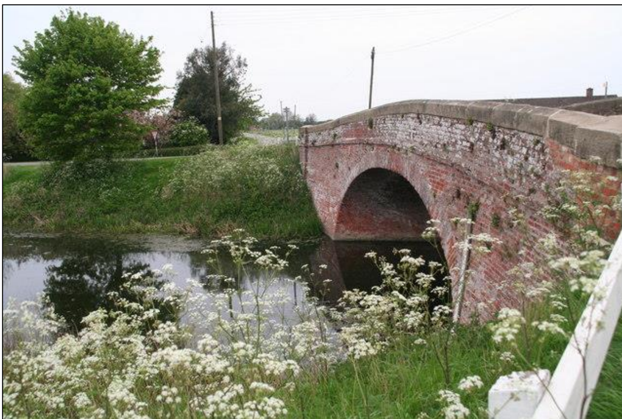
Figure 3: East and West Fens at Stone Bridge Drain
