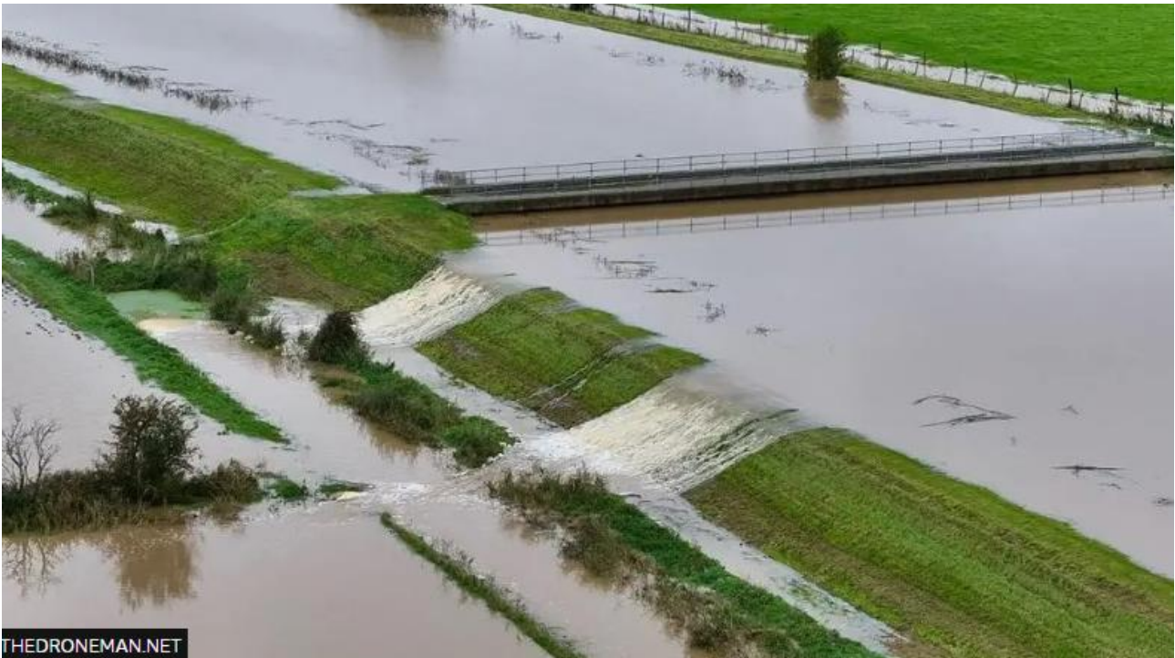
Figure 20: Overtopping of Steeping River relief channel
