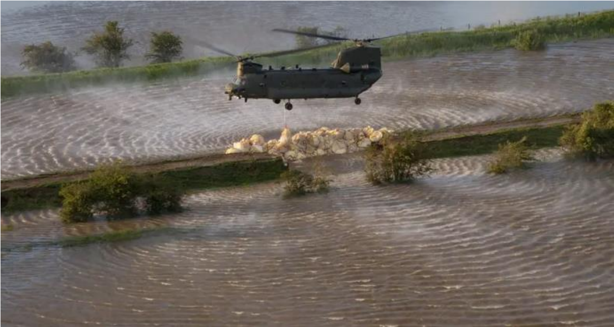
Figure 13: RAF helicopter dropping ballast to plug the breach 24
