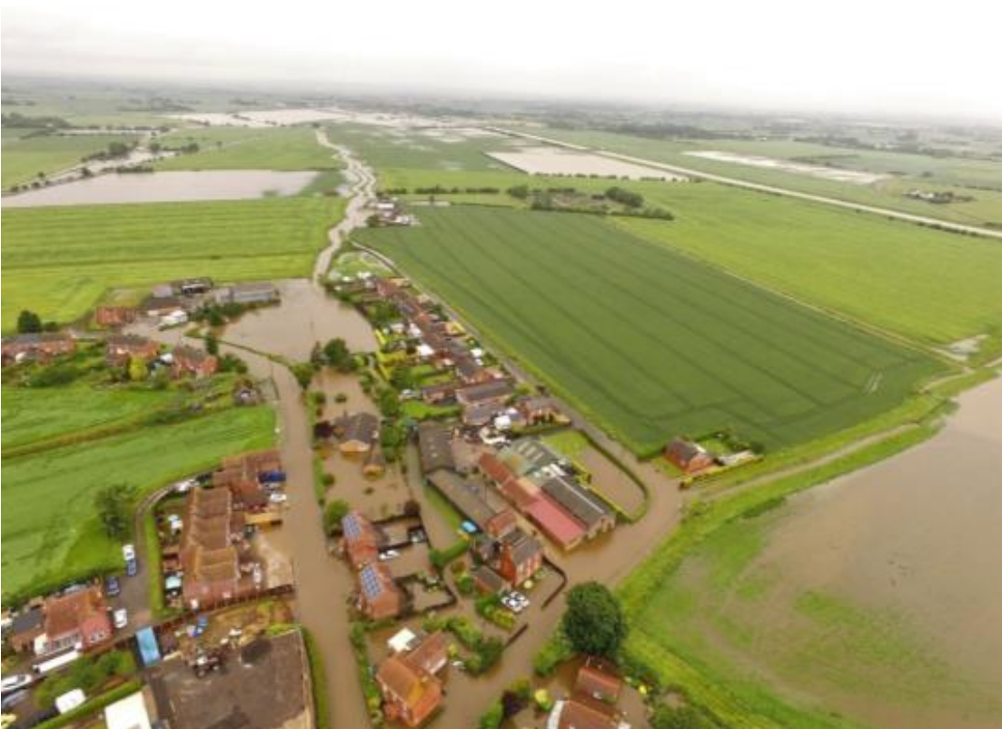
Figure 12: Flooding at Wainfleet (c) Lincolnshire Community Council
