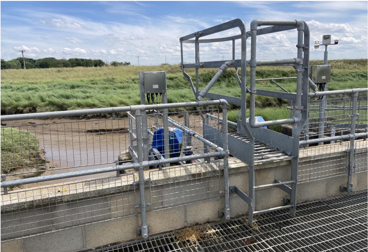
Figure 5: Burgh Sluice © Arup
