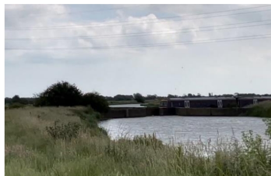
Figure 3: Railway crossing and sluice of the Wainfleet Relief Channel © Sam Hazell
