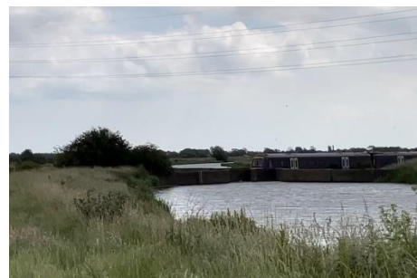
Figure 11: Photograph 1: Railway crossing and sluice of the Wainfleet Relief Channel © Hazell, N.D
