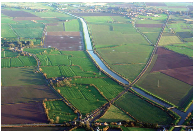
The Wainfleet Relief Channel, showing the crossing of the Boston to Skegness Railway Line © Chris. Licensed for reuse under the Creative Commons Licence
