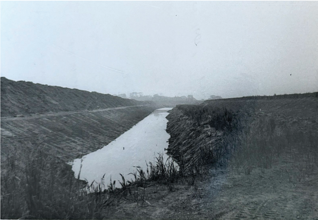
Construction of the Wainfleet Relief Channel © Environment Agency
