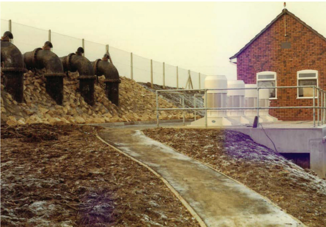
Construction of the new Thorpe Culvert Pumping Station © Anglian Water 1982
