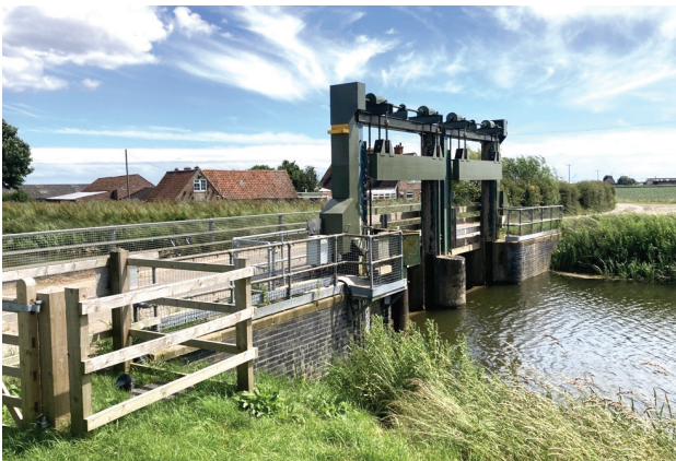
Haven House Sluice © Arup 2024
