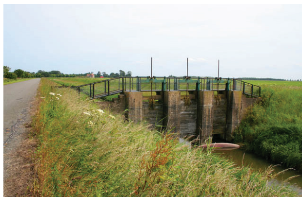
Sluice on the Cow Bank Drain
