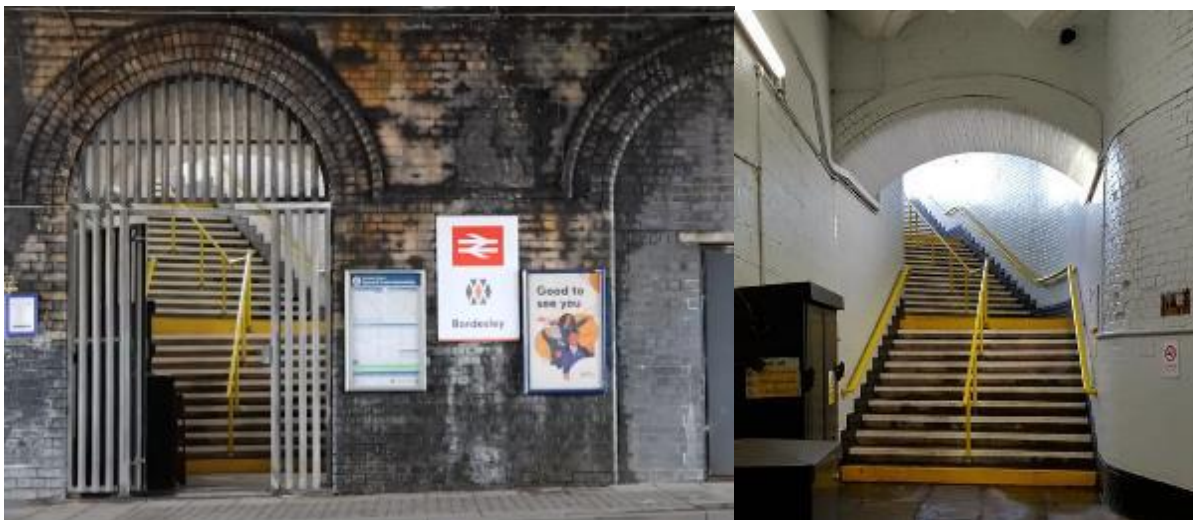
Figure 6: (left) Bordesley station entrance from Coventry Road showing start of staircase access to platforms and (right) closer view of staircase access to platform level
