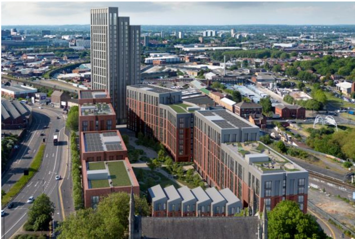
Figure 11: Visualisation of Smith's Garden development currently under construction with Bordesley station platform on the lower right and the proposed site of the Bordesley West Chord to the right of the development at the bottom right of the image
