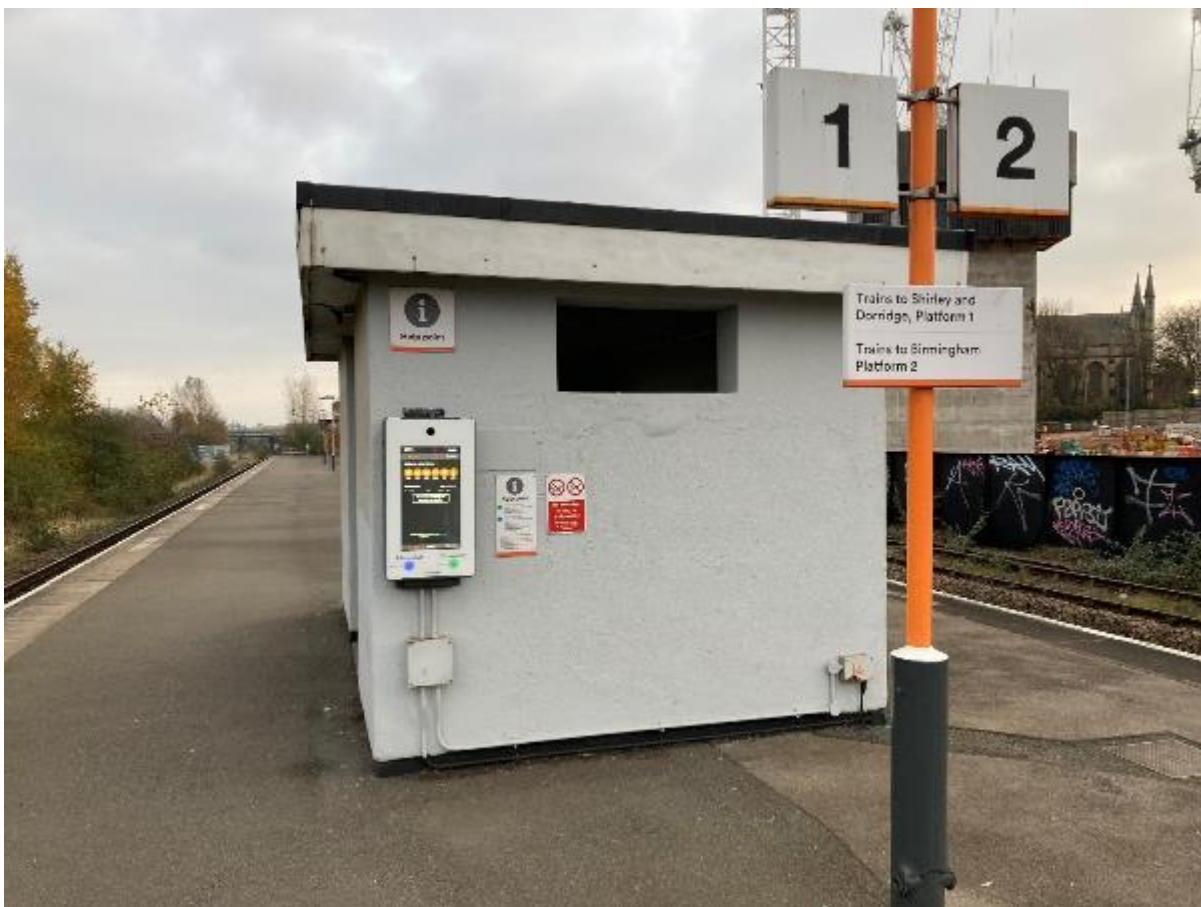
Figure 4: Bordesley station platform, shelter and Help Point / Information Screen
