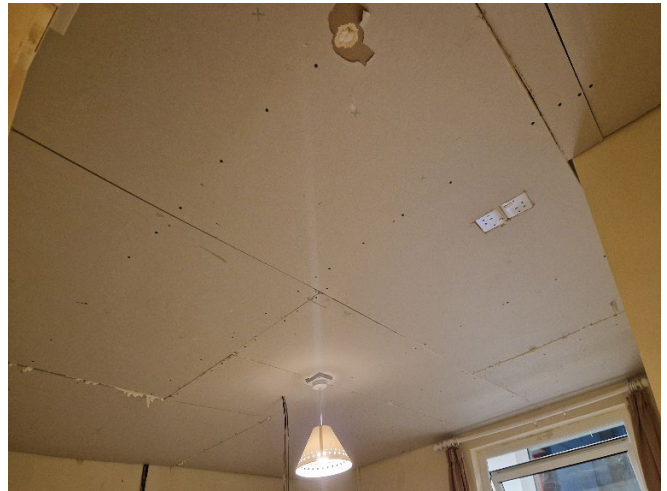
Figure 2-9 IR Heater type 6 installed in Room C (mid-install left, covered pre-plaster right)
