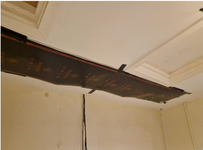
Figure 2-9 IR Heater type 6 installed in Room C (mid-install left, covered pre-plaster right)
