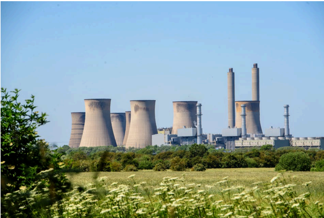
Figure 7 – The West Burton site before STEP construction
