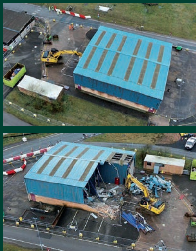
'Before' and 'during' shots of the demolition
