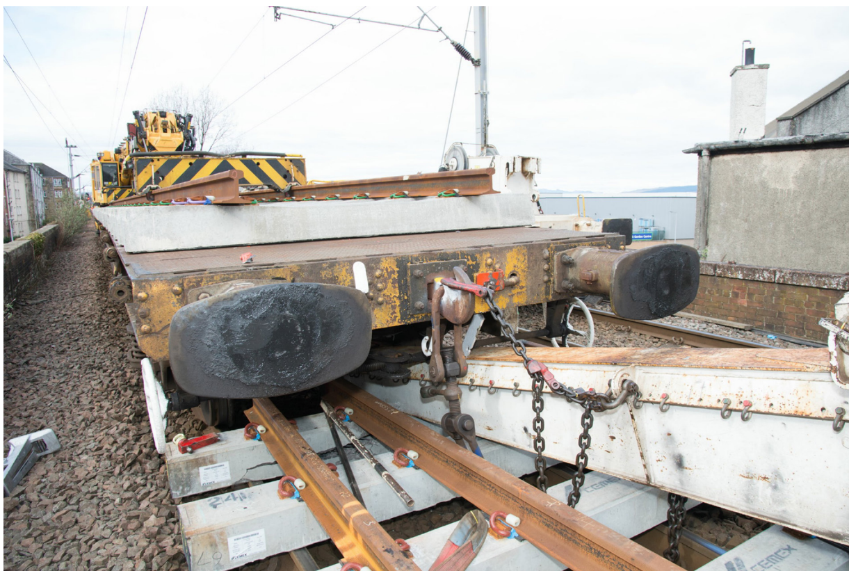
Figure 17: The end of the salmon wagon, after the collision, showing no lighting fitted (courtesy of British Transport Police; taken after two of the panels had been removed).
