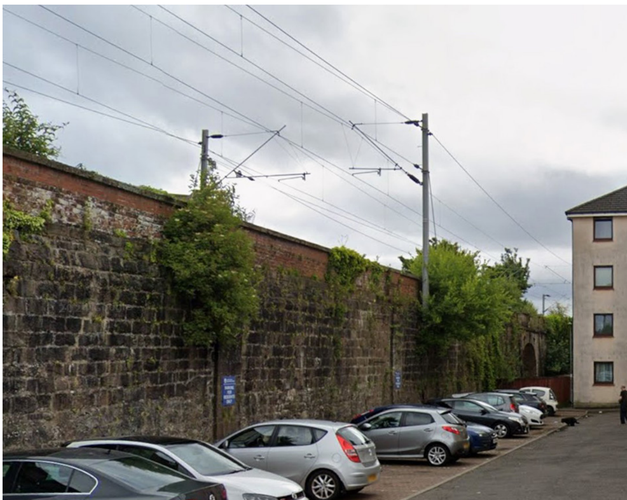
Figure 4: Raised structure at the accident location.
