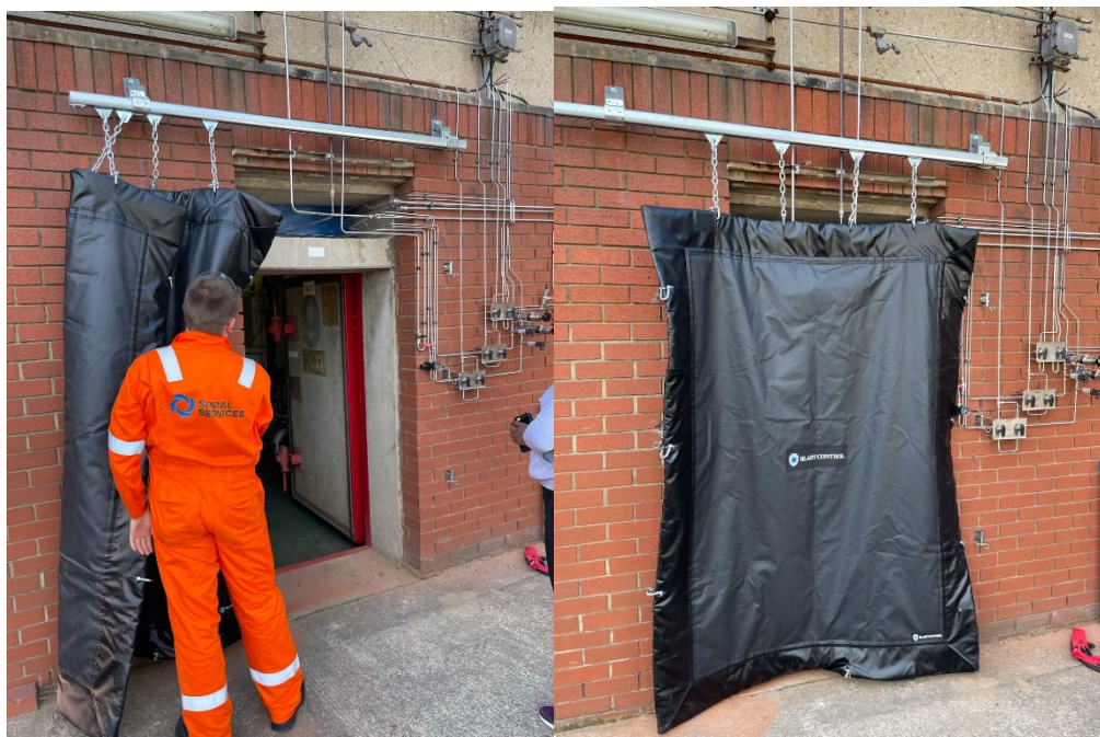
Figure 11 - Blast bay curtain being installed outside Bay 9 door.
