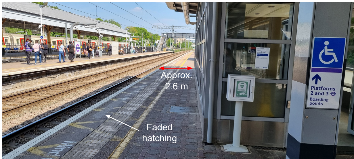
Figure 15: The waiting room and narrowest point close to where the trap occurred.
