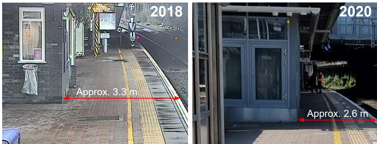
Figure 17: Old waiting area building (taken in 2018) and the new building (taken in 2020) (courtesy of Network Rail).
