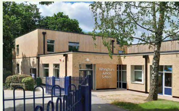
This project piloted an innovative approach to the retention and recladding of an occupied 1960s system-built junior school, through the development of an offsite-manufactured structural timber replacement external envelope.
