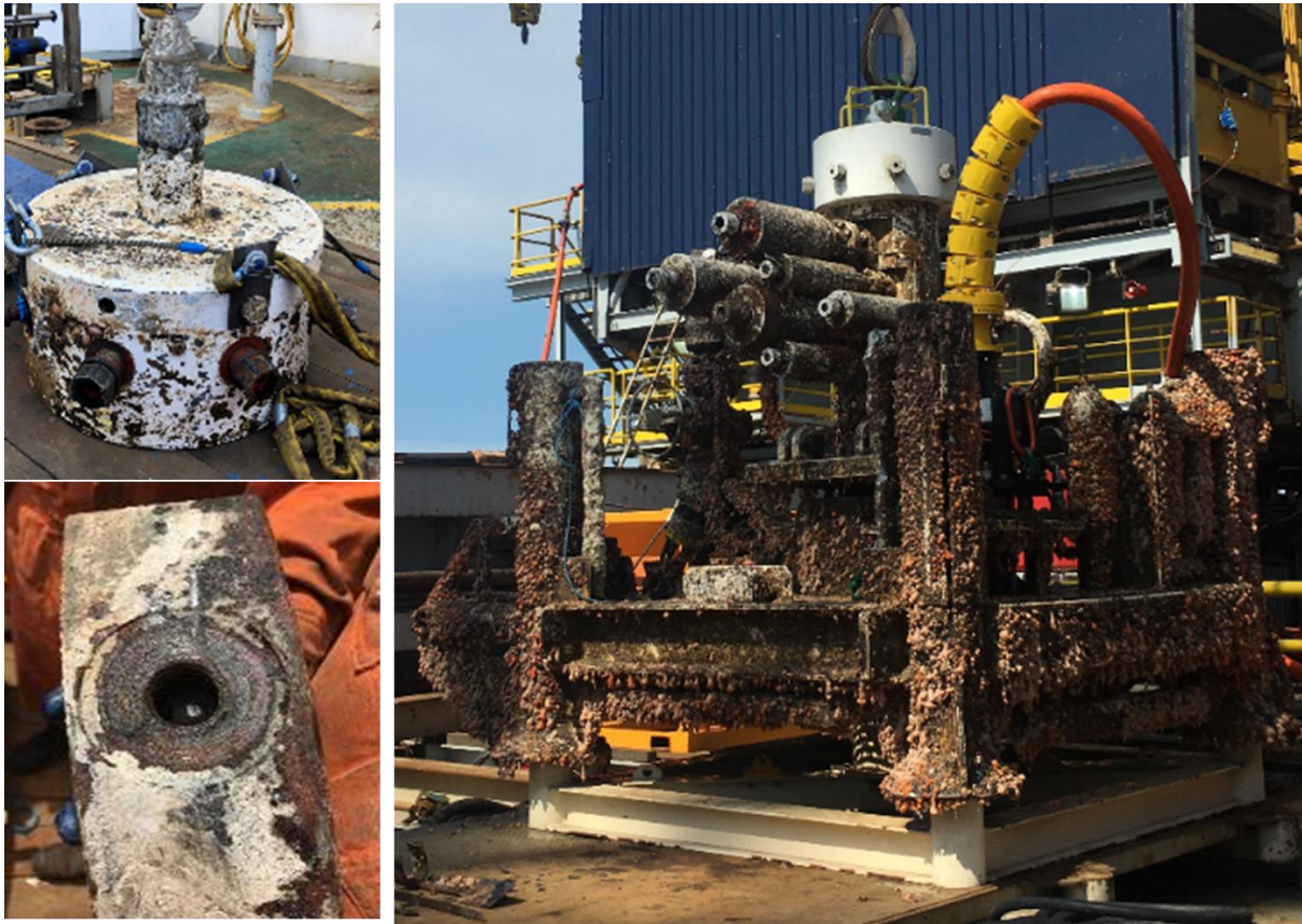
Figure 8.4 – Removal of Bure Oscar subsea wellhead onto barge
