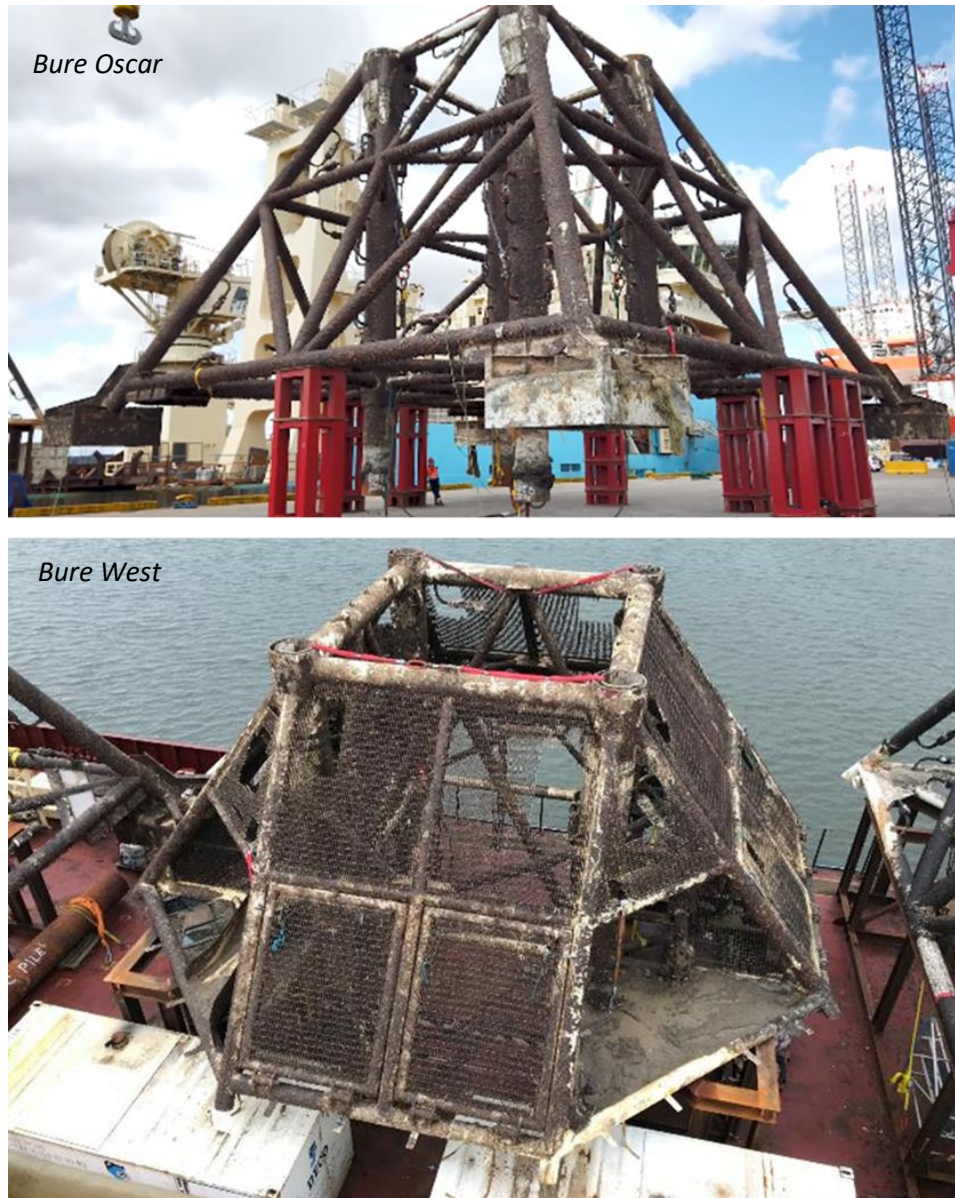
Figure 8.5 – Set-down of Bure Oscar subsea protective at Port Blythe yard & Removal of Bure W subsea protective cage onto the barge.
