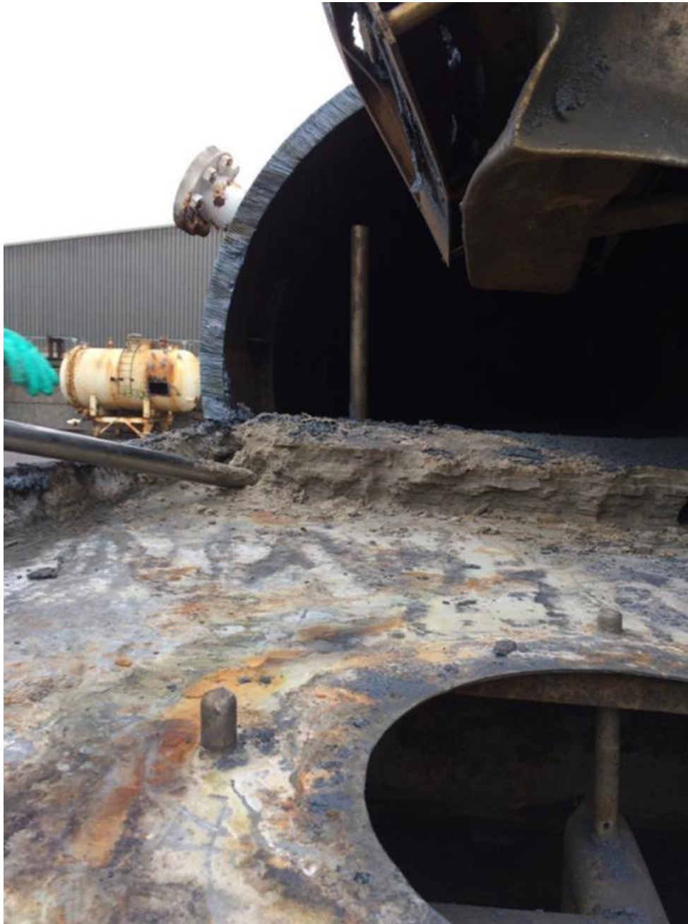
Figure 8.3 – Removal of NORM contaminated sand from Thames process vessel at Hoondert Yard
