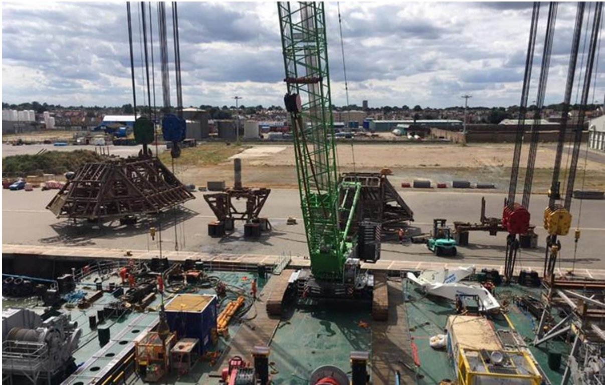
Figure 8.6 – Set down of Thurne WHPS structure (behind crane) on the quayside at GY Veolia yard.
