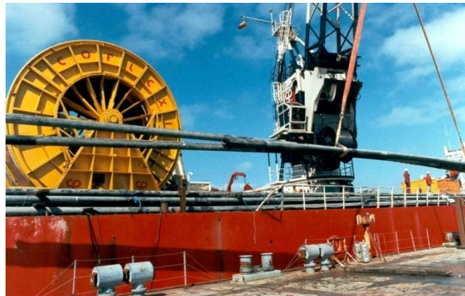
Figure 3-4: Pipeline Cut into Section for Recovery
