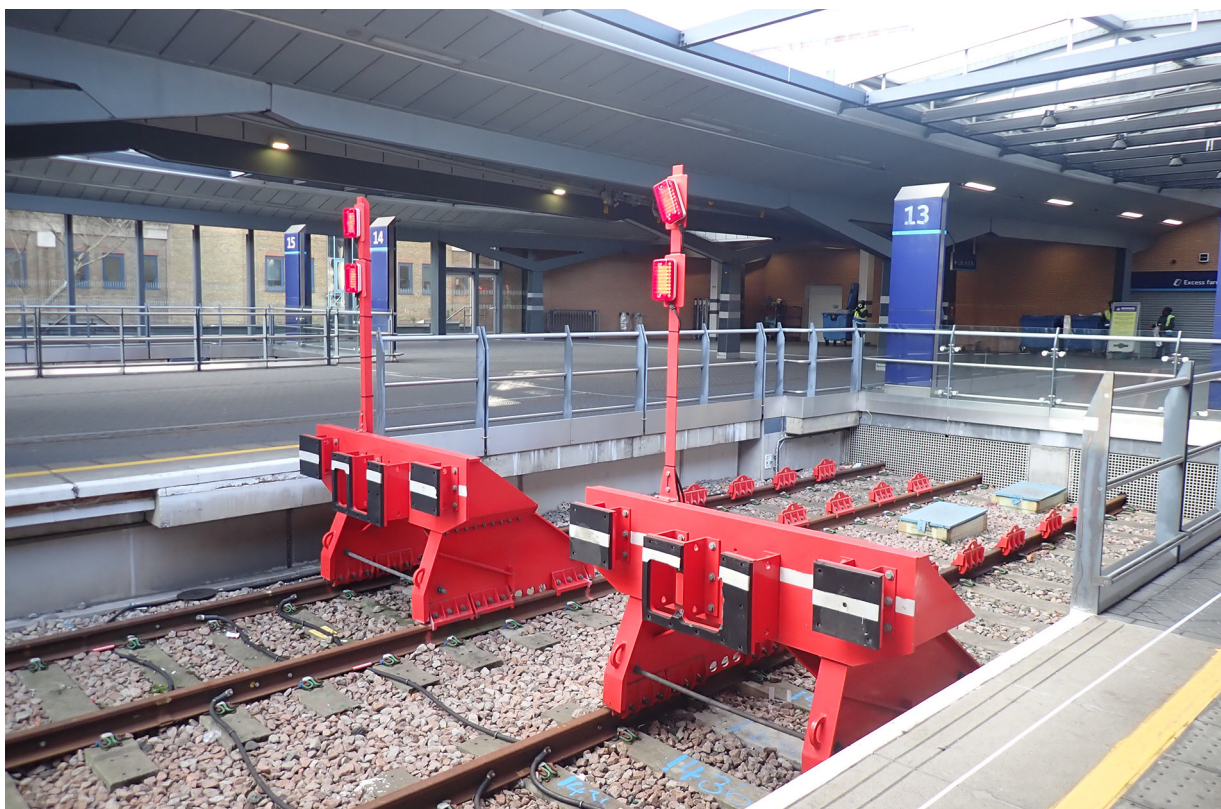
Figure 4: On the right, in their normal position the buffer stops of platform 12 at London Bridge station (courtesy of Network Rail).
