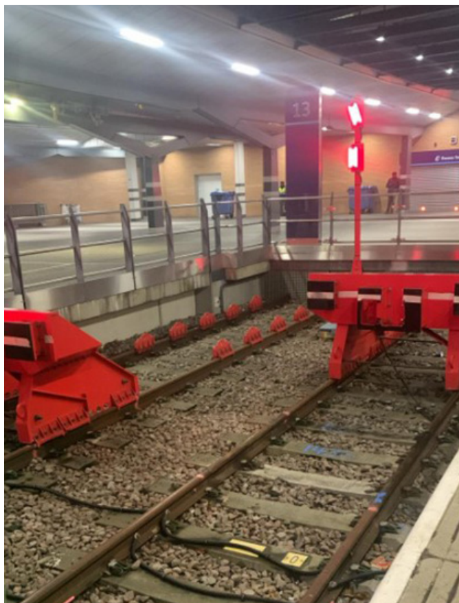
Figure 6: Buffer stops at London bridge platform 12 after the collision.
