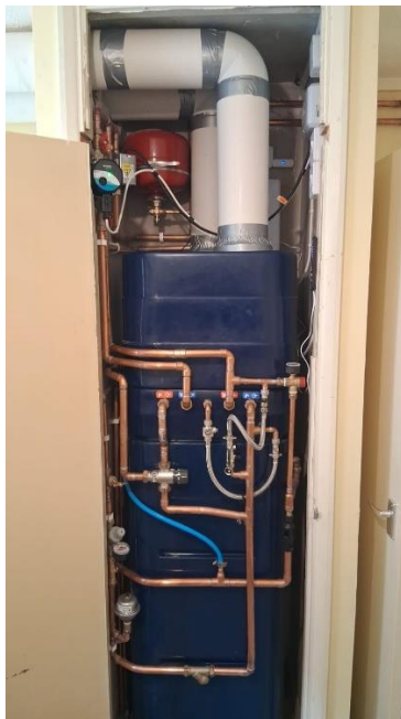
Figure 1: CUBEX installation in a narrow airing cupboard
