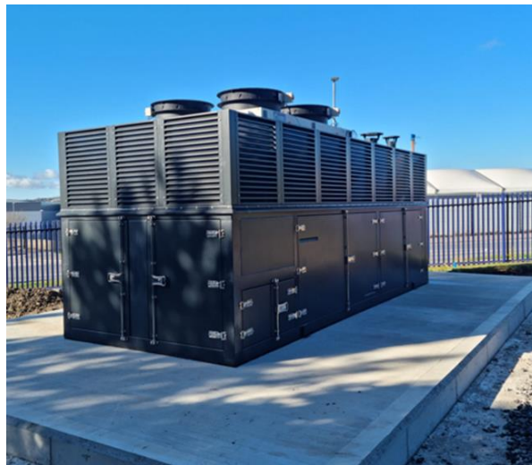
Figure 1: An illustration of Vital Energi's 'Therma Hub' heat pump solution sited outside the building
