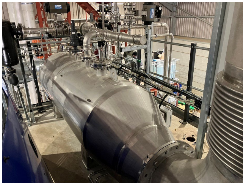
Figure 18 - Air-to-steam generator
