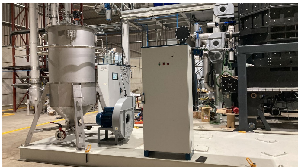
Figure 21 - Flue Gas Scrubber
