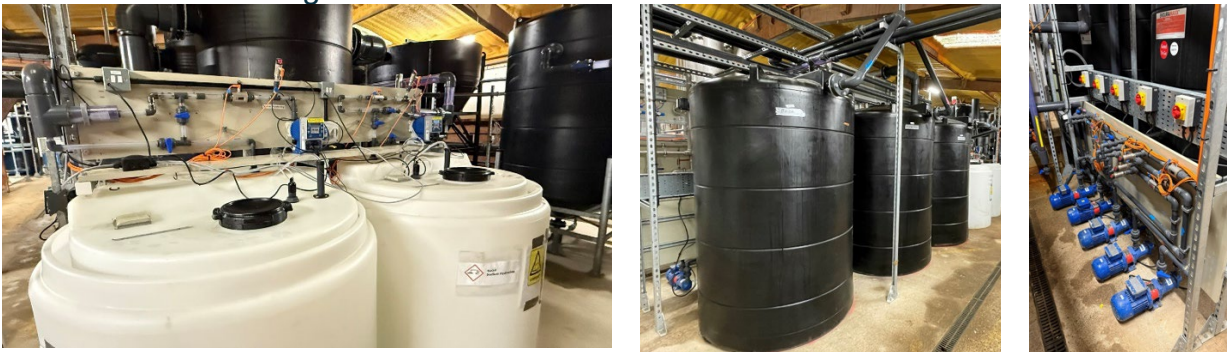
Figure 12. Two of the bunded bulk chemical tanks and a dosing station, BPMED acid, base and desalinated water product tanks, BPMED product dosing pumps.
