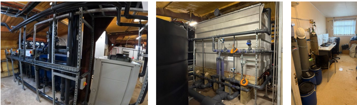
Figure 11. Blowers and air intake (and outflow) pipework, Seawater CO 2 stripper and break tank & CO 2 monitoring system.
