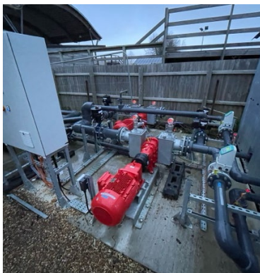
Figure 9. Seawater extraction skid, intake and outflow pipework crossing Site & intake and outflow entering plant.
