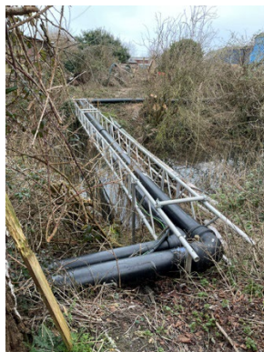
Figure 9. Seawater extraction skid, intake and outflow pipework crossing Site & intake and outflow entering plant.
