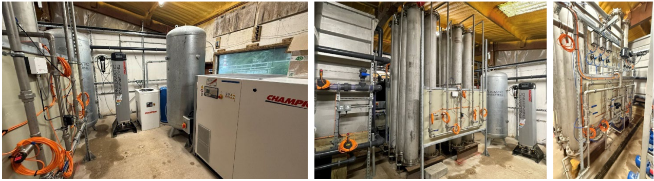
Figure 13. Compressor, receivers and dryers.
