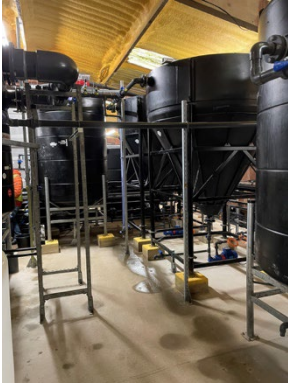
Figure 10. Seawater pre-treatment precipitation and settling tanks, BPMED unit and cell.
