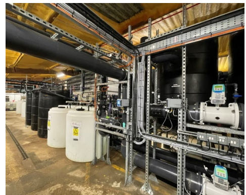
Figure 9. Seawater extraction skid, intake and outflow pipework crossing Site & intake and outflow entering plant.
