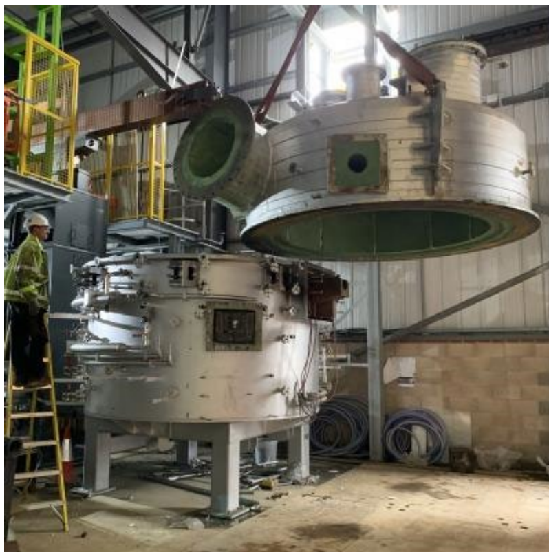
Figure 38 – Lifting Plasma Furnace Roof into Place
