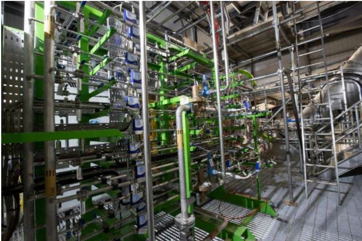
Figure 22 – Carbon Dioxide Distribution Manifold
